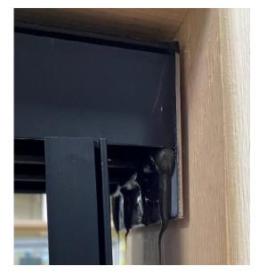
2.J. On the exterior side, measure the frame opening height at each jamb and cut a board to use as a gauge/guide to help level the head to the height of the frame opening at the jambs. Position the gauge board in the frame at each installation screw hole location to confirm the frame
