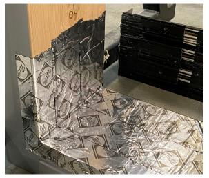
1.D. Position the door sill into place. Mark the interior sill edge (full length), sill ends, and prepiloted anchor locations. Sill anchor pilot holes will be located in interior and exterior tracks (and middle track on a five-track frame) under the weatherstrip approx. 4" from each end and 18" OC.
