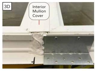
E. Cover exposed joint with flashing tape. Make sure the tape closely follows the contours of the frame profile.
