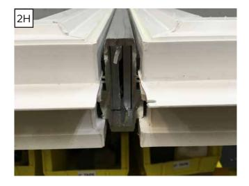
Outline each end of the mullion reinforcement with sealant ensuring the sealant touches off on all 4 ends of tape pieces.
