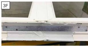
G. Clean any excess sealant squeeze-out with Isopropyl Alcohol and a rag.
