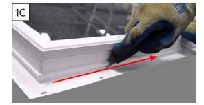
D. **Bend the fin down and then up** to remove the fin from the frame.
