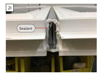
J. **Install a foam plug** on each end of the mullion against the sealant.
