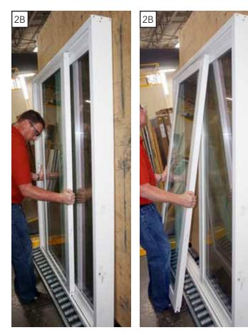
C. Place the panel on edge to gain access to the roller attachment screws.
