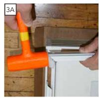
B. Place each jamb clad piece onto the cornerlock. Insert a cornerlock screw through the frame head into the cornerlock.
