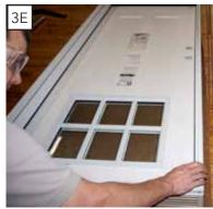
F. Starting on one head and jamb corner; use a block of wood and mallet to tap the frame clad onto the molded nose.
