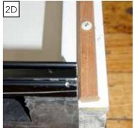
E. Continue drilling pilot holes on 8" centers along the length of the molded nose.
