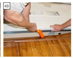
C. Fold out the fin to 90°. This fin is to be used for **flashing only** not for installation.
