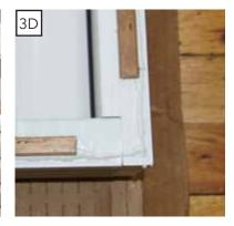
E. Position the assembled clad frame over the molded nose.
