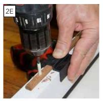
F. Insert a screw into each pilot hole.
