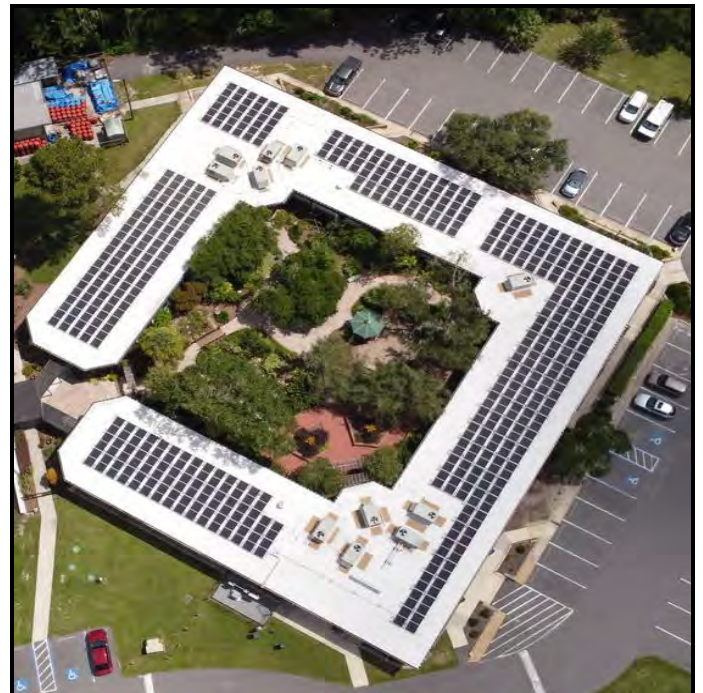
Solar Panels – Cooperative Extension Office
