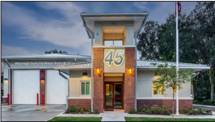
Central Brandon Fire Station #45
