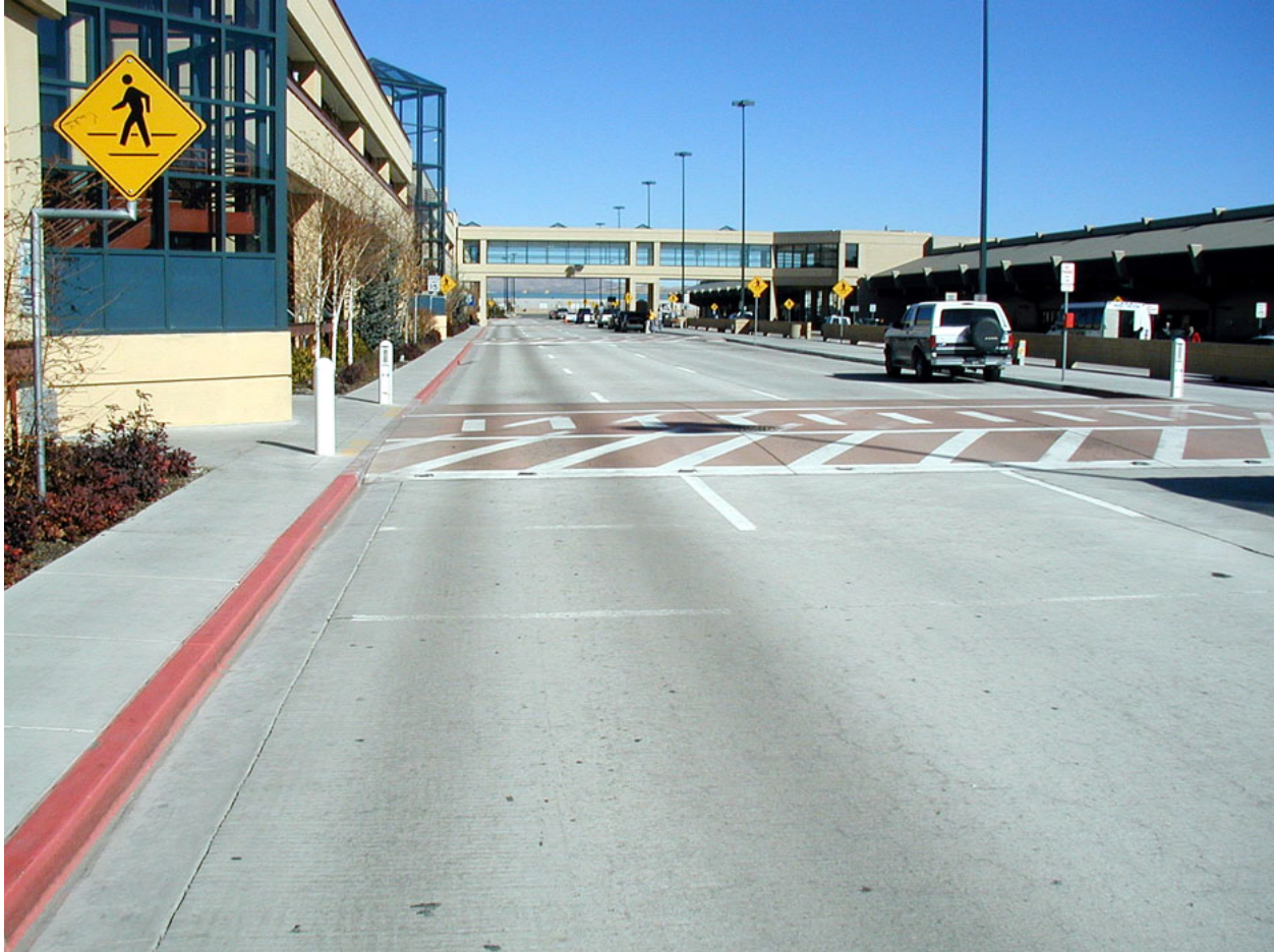
Figure 21: A raised crosswalk with brick paver treatment in Reno, NV. Source: pedbikeimages.org /Dan Burden
