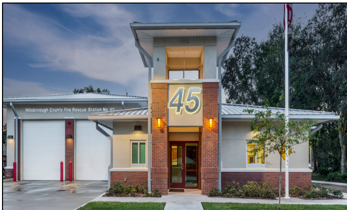
Central Brandon Fire Station #45
