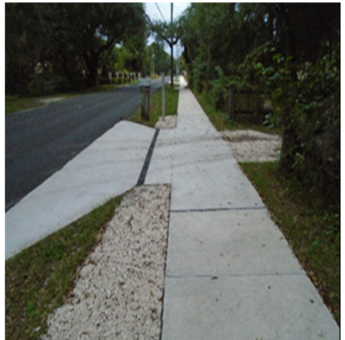
Sidewalk Repair Program
