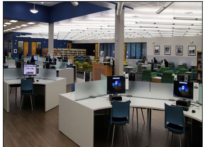
North Tampa Library Renovations
