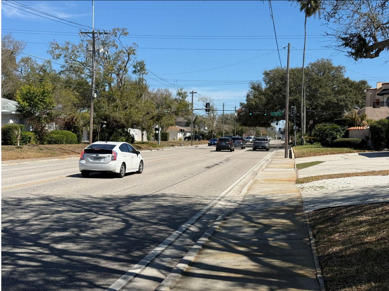
Figure 4: Eastbound Bay to Bay Blvd at Church Ave, Showing Oak Tree Over the Eastbound Signal Mast Arm
