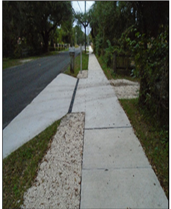
Sidewalk Repair Program
