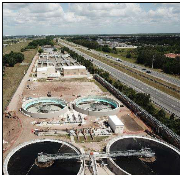
South County AWWTF Modular Expansion
