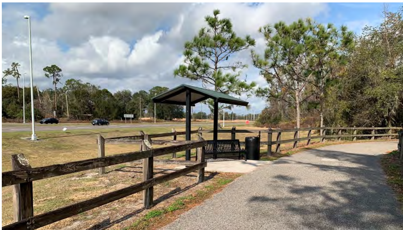
Figure 28. – Wayside designed with shade structure and separation from the roadway
