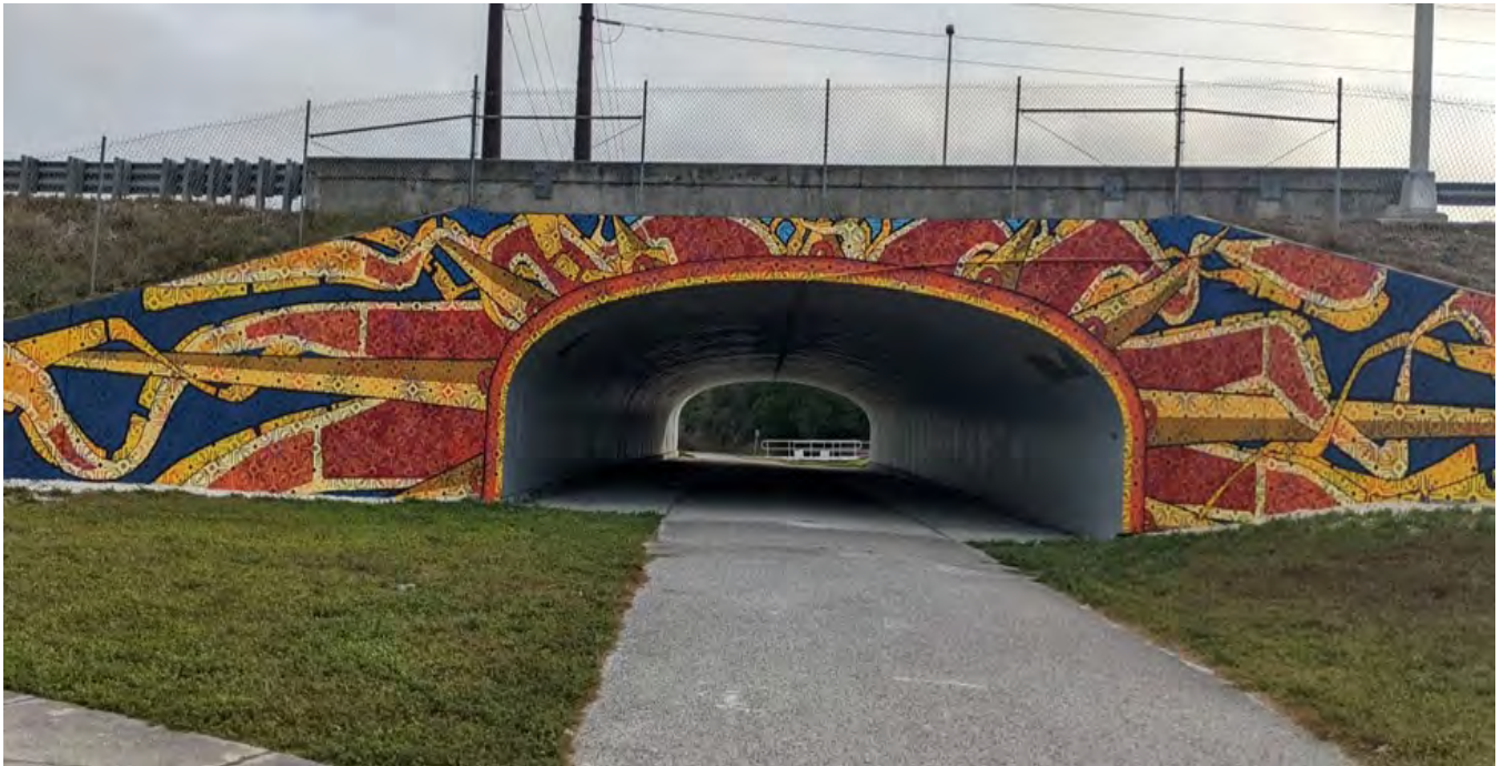
Figure 25. Underpass with public art enhancement and width to enhance natural lighting and safety
