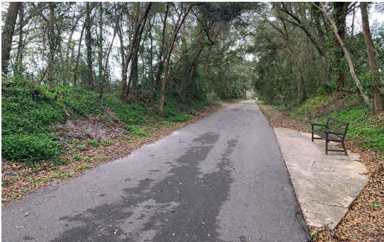
Figure 27. Wayside with contrasting surfaces and furniture set back from pathway edge
