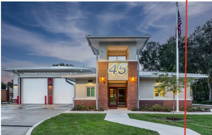
A community of over 116,000 residents and hundreds of businesses now has a new, modern fire station calling Central Brandon home.
