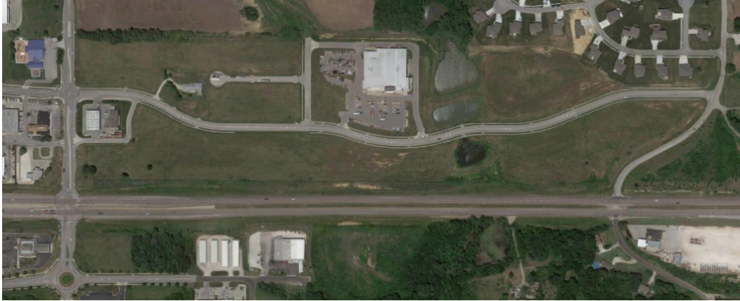
Figure 36. Service road funded by KDOT access management set-aside funds.
