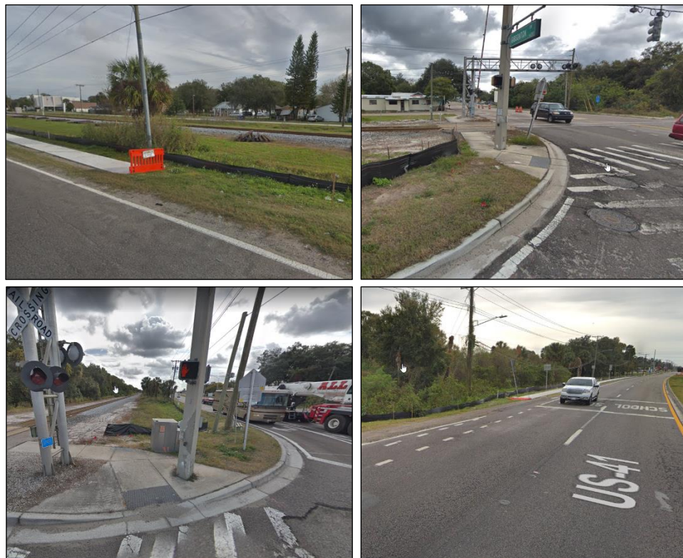
Figure 31. Sidewalks under construction on US 41
