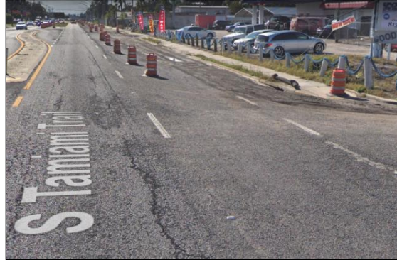
Figure 36. Construction on US 41
