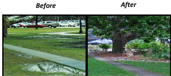
Rain Garden System
