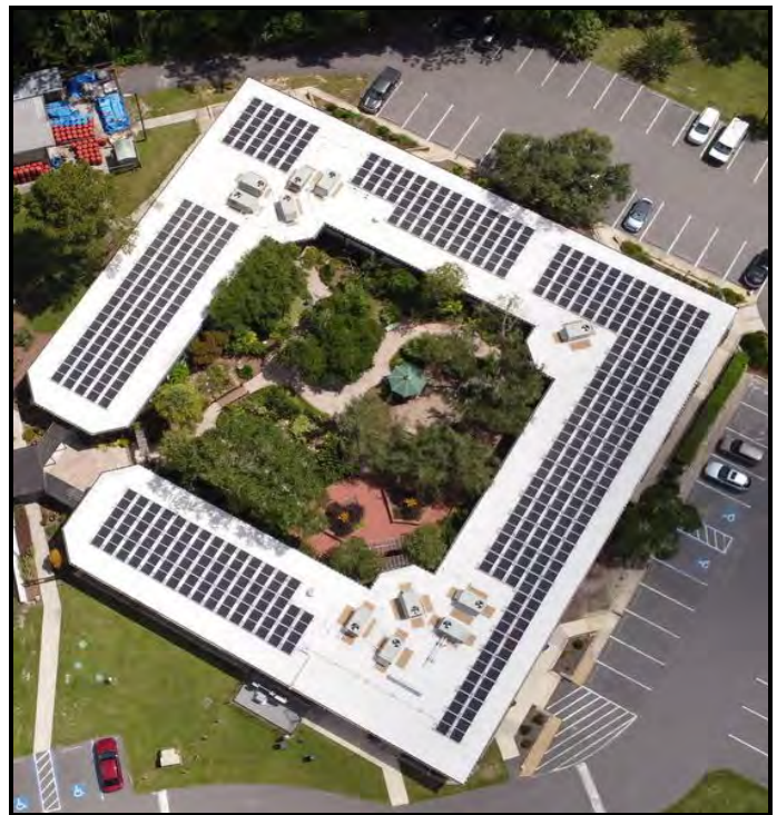
Solar Panels – Cooperative Extension Office
