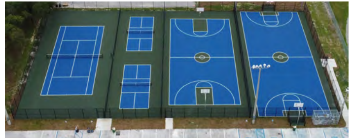
R3M replaced the tennis courts with a new multipurpose court at Town & Country Park as part of lifecycle replacement.
