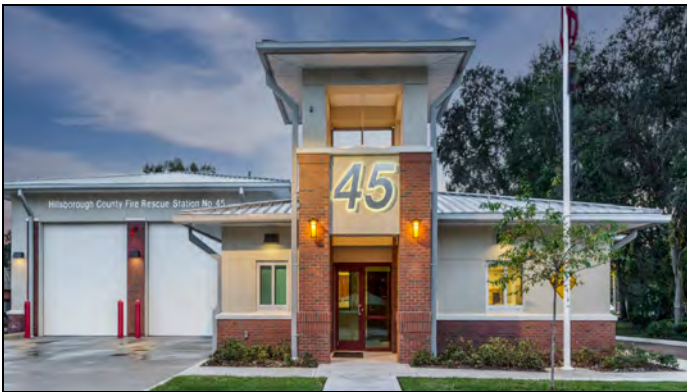
Central Brandon Fire Station #45
