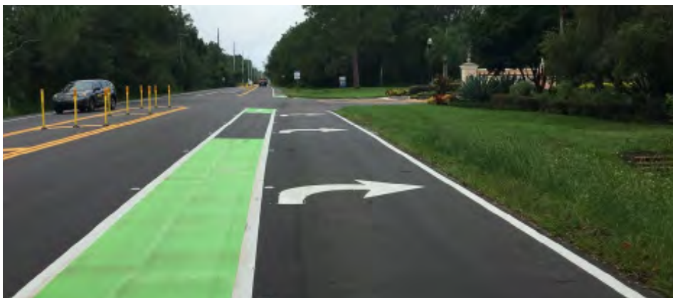
Cory Lake Boulevard was resurfaced, and the right of way was used to create a right-turn lane to reduce rear-end collisions and congestion.
