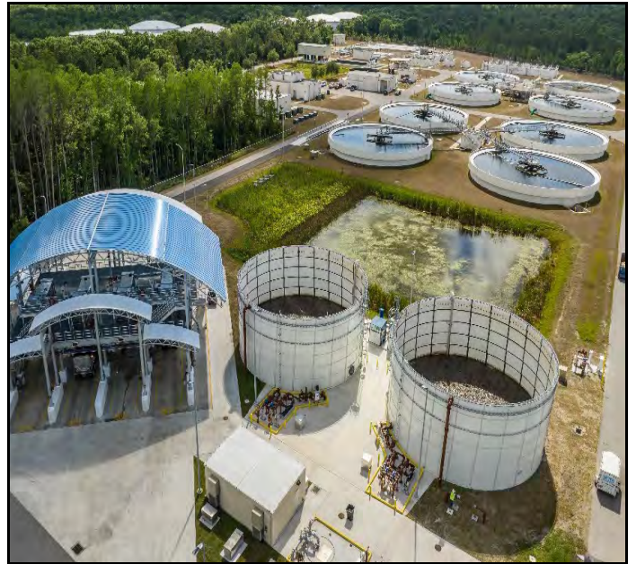
Northwest Regional Water Reclamation Facility System Improvement & Expansion
