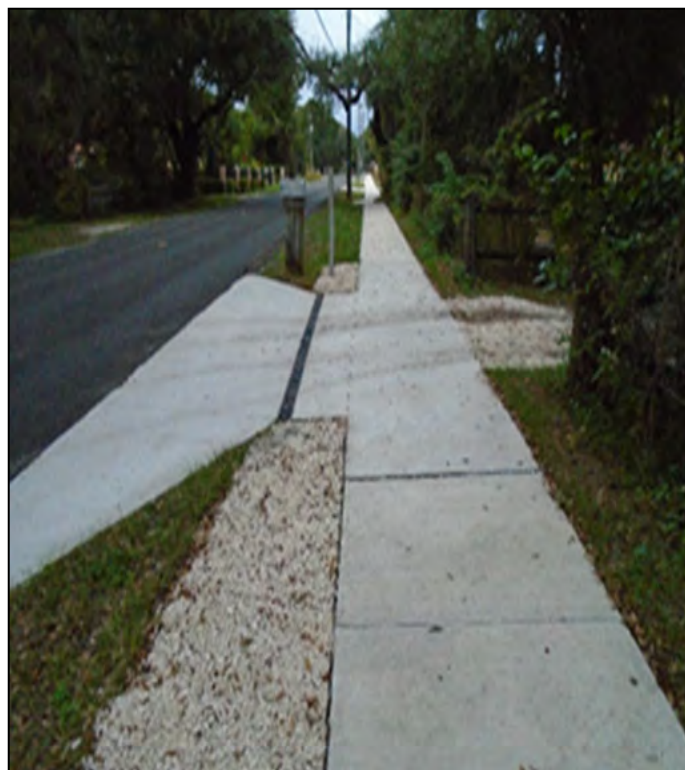
Sidewalk Repair Program
