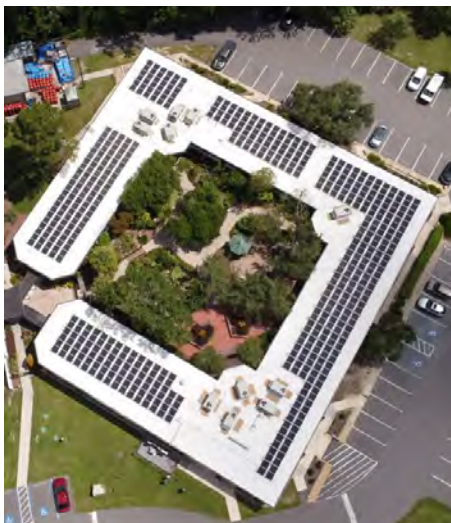
R3M installed a 122kW solar panel system on the roof of the Cooperative Extension Office for continued sustainability efforts.
