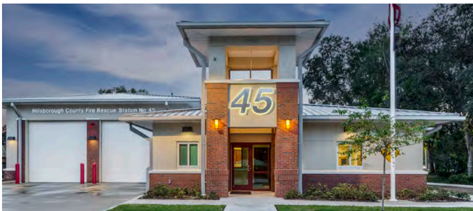
Fire Rescue opens Fire Station #45 in Central Brandon.
