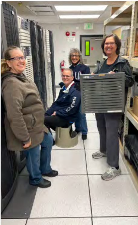
Information Technology staff decommissions a 20-Year-Old CLASS Server.
