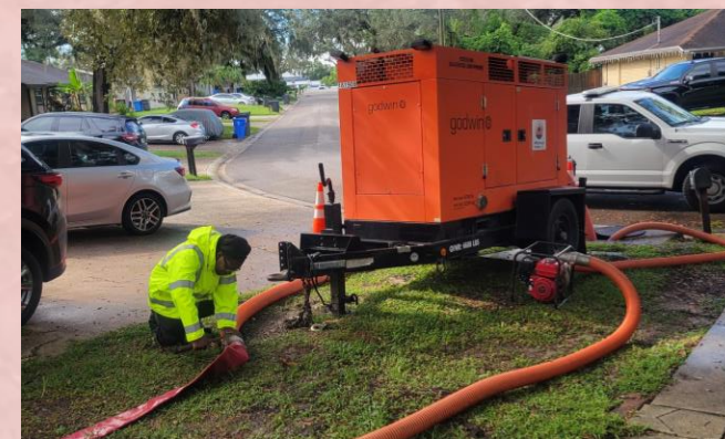
Pump Station Restoration
