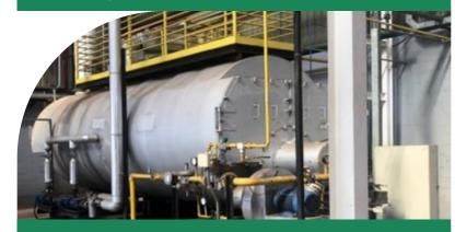
At our Senador Canedo site, we continue to operate a biomass boiler powered by old and damaged wood pallets.
