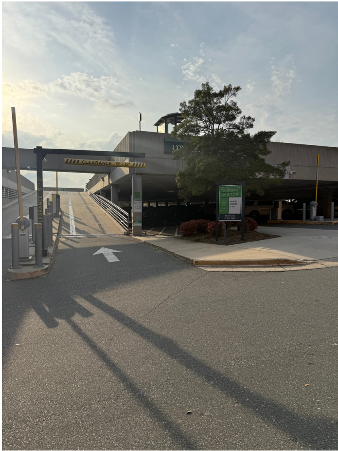
Cone Deck Rooftop
