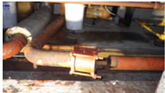
Photo 8: Separated brine system coupling.
