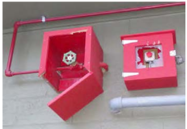
Photos 16 (left) and 17 (right): Opened Emergency Discharge Valve and Actuated Emergency Stop Button.
