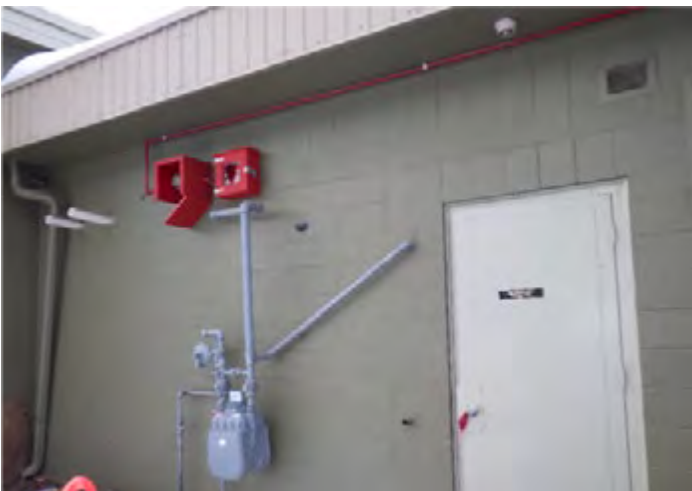
Photos 16 (left) and 17 (right): Opened Emergency Discharge Valve and Actuated Emergency Stop Button.
