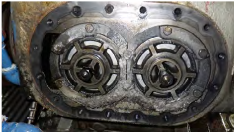
Photo 7: Build-up of salt crystals from brine around lower compressor cylinder heads of compressors #1 and #2.
