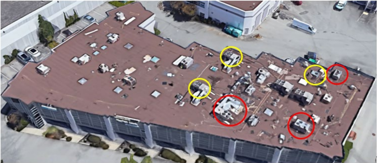
Image 7 (2022) - Rooftop/air conditioner units added 2002 to 2014 (yellow) and 2014 to 2017 (red)
