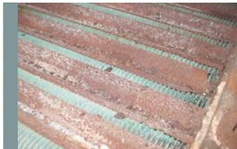
PLUGGED AND CORRODED BOILER HEAT EXCHANGER
