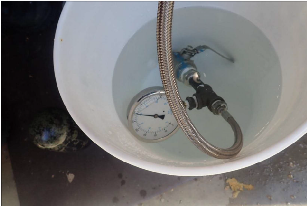
Figure 12 Typical leak test @ 200 psi.
