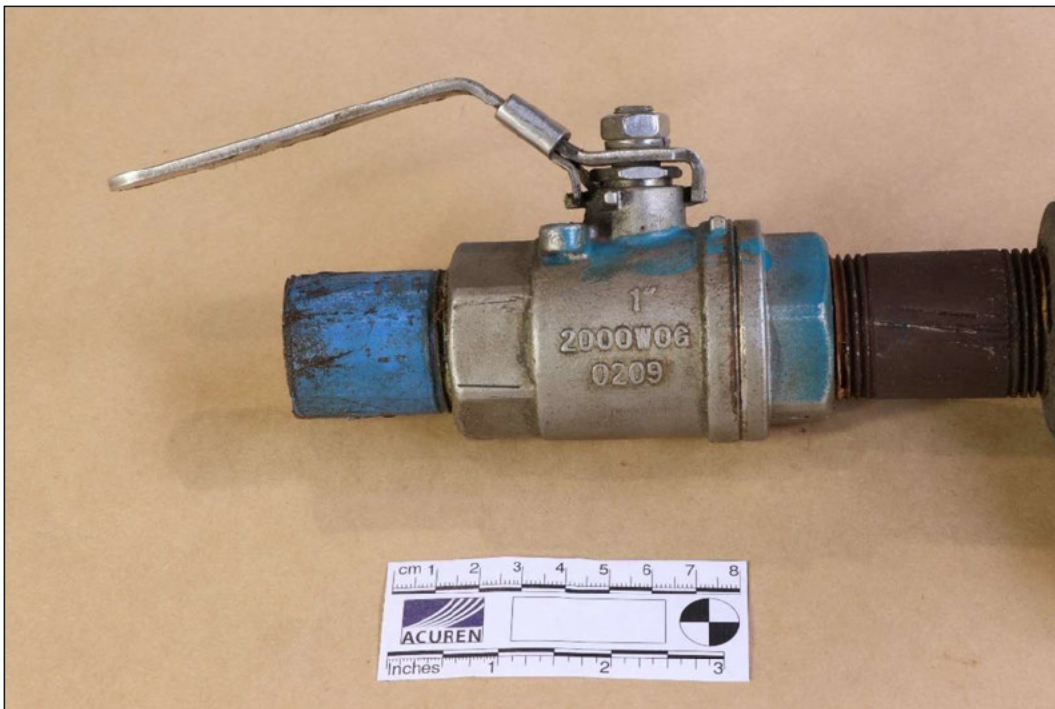
Figure 3 View of valve showing downward permanent bend in lever of approximately 20°.
