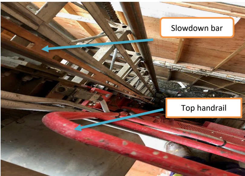
Slowdown bar mounted to bracket which attaches to mast.
