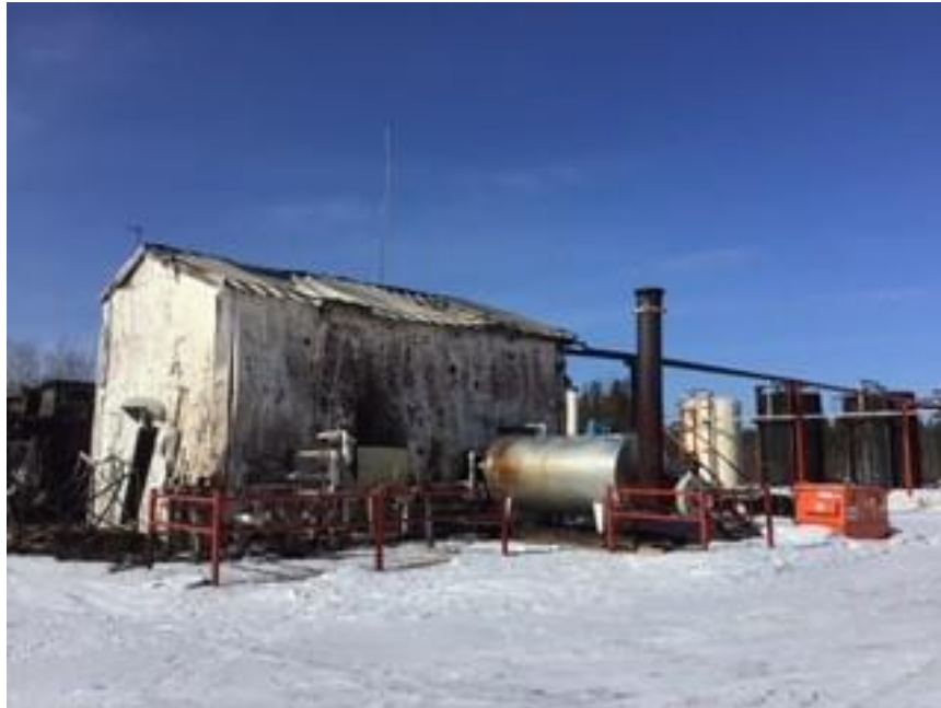
Looking from South East End of facility
