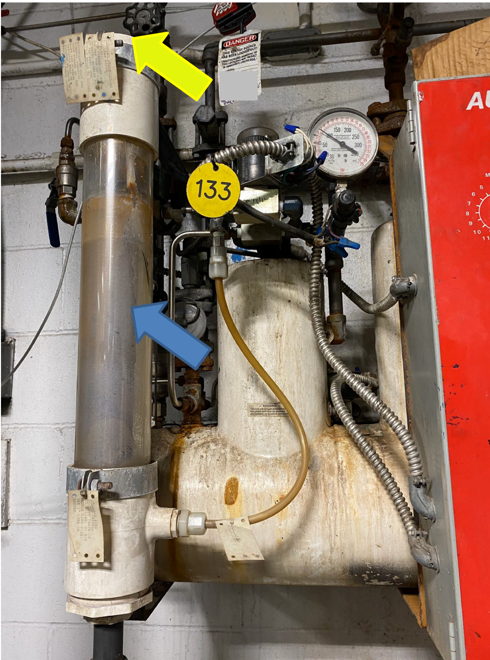
Image 3 – Blue arrow indicating water bubbler tube. Yellow arrow indicating location the water bubbler tube cap should be installed.
