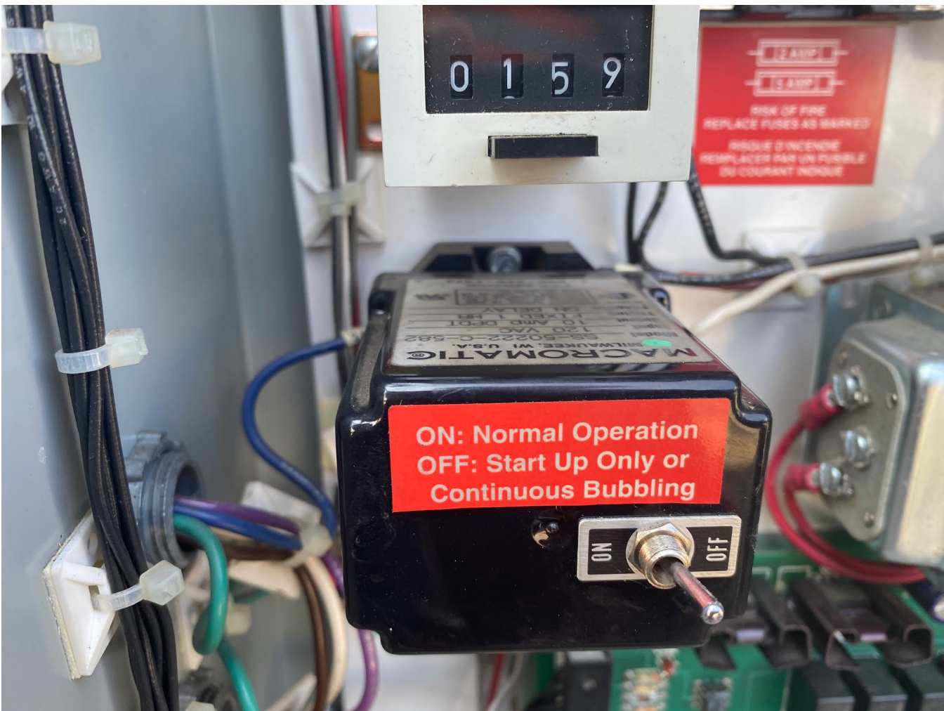
Image 6 – Auto purger time delay relay switch as found in the “Off” setting for startup or continuous bubbling. In this position the auto-purger would not shut the purge solenoid if it purged for longer than 60 minutes. If set to normal operation the purge solenoid would have deactivated after 60 minutes possibly reducing the amount of ammonia released.
