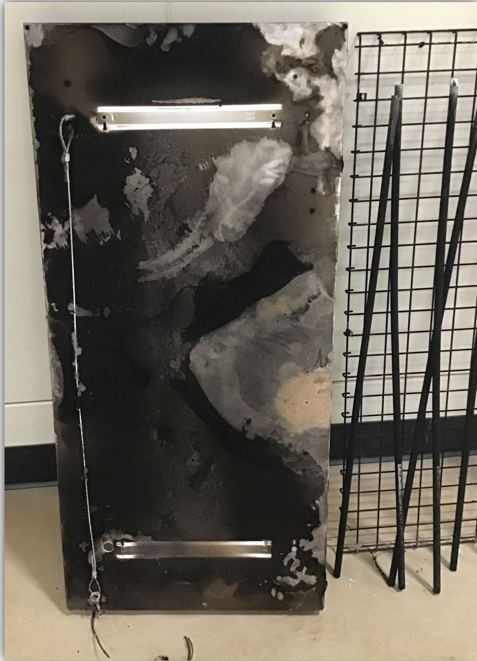
Image 3 - Damaged luminaire, tubes, and cage – note that the polymer lens had completely melted away.
