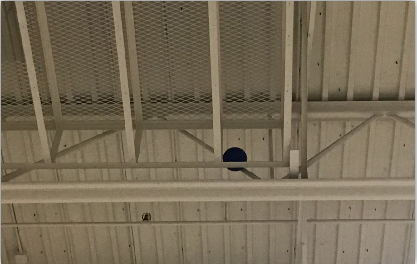
Image 5 - Example of balls kicked up and wedged to ceiling system.
