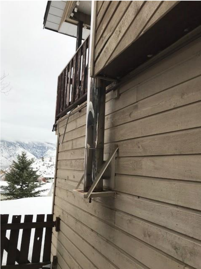
Bottom section of vent and chimney base tee
