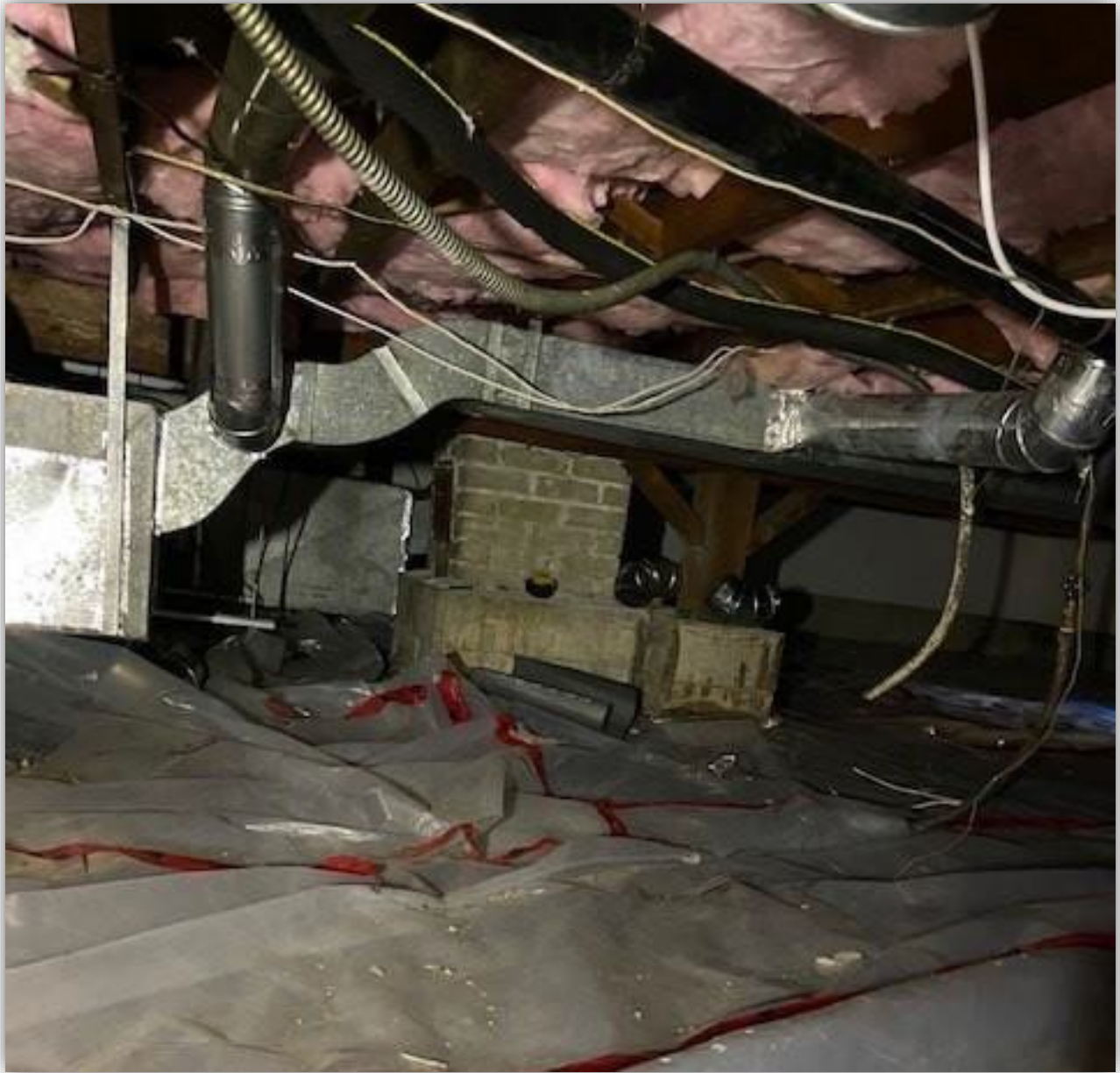
Image 2 - Crawl space where incident occurred.
