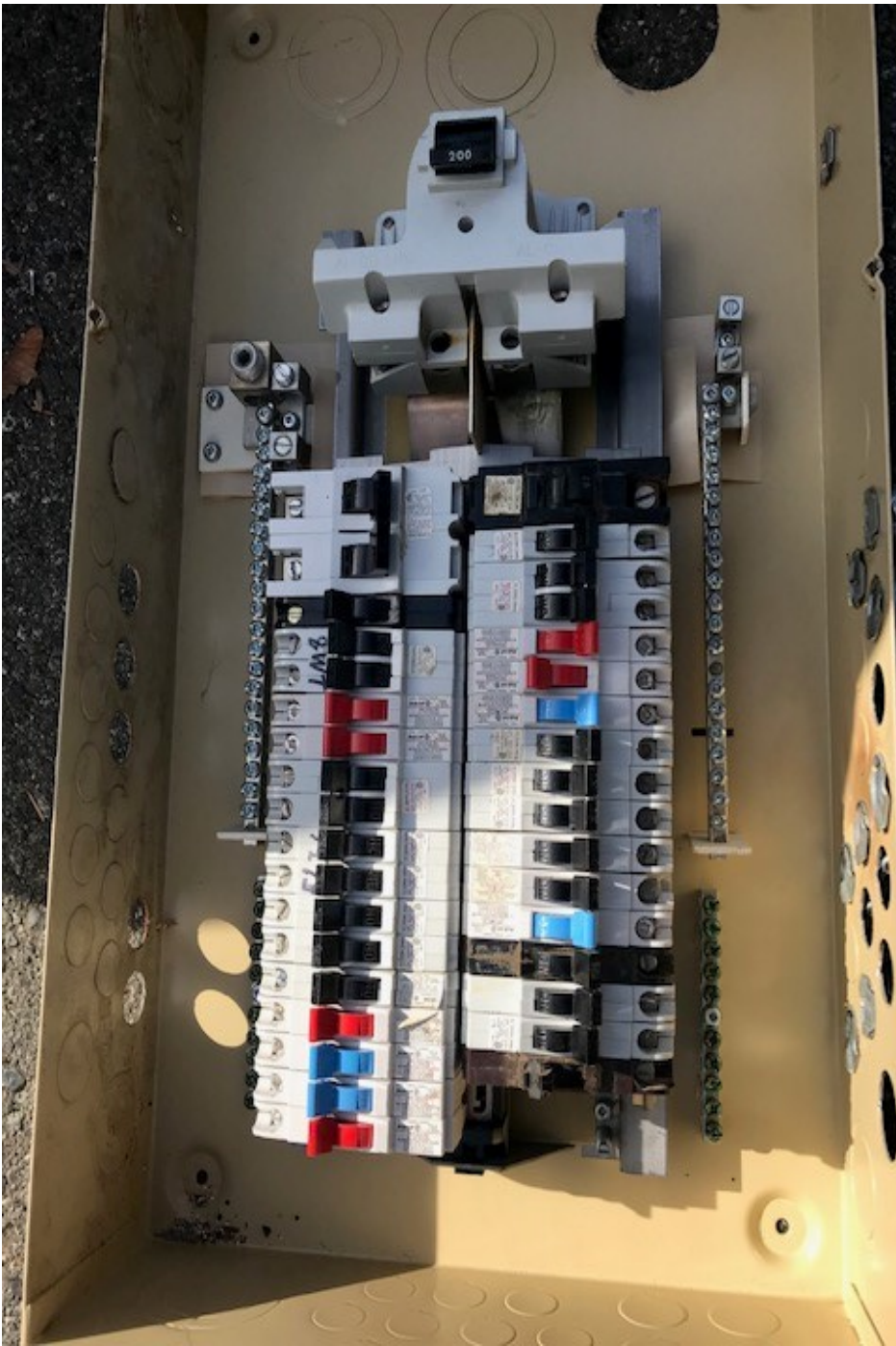
Photo 1: FPE 200A breaker panel removed
