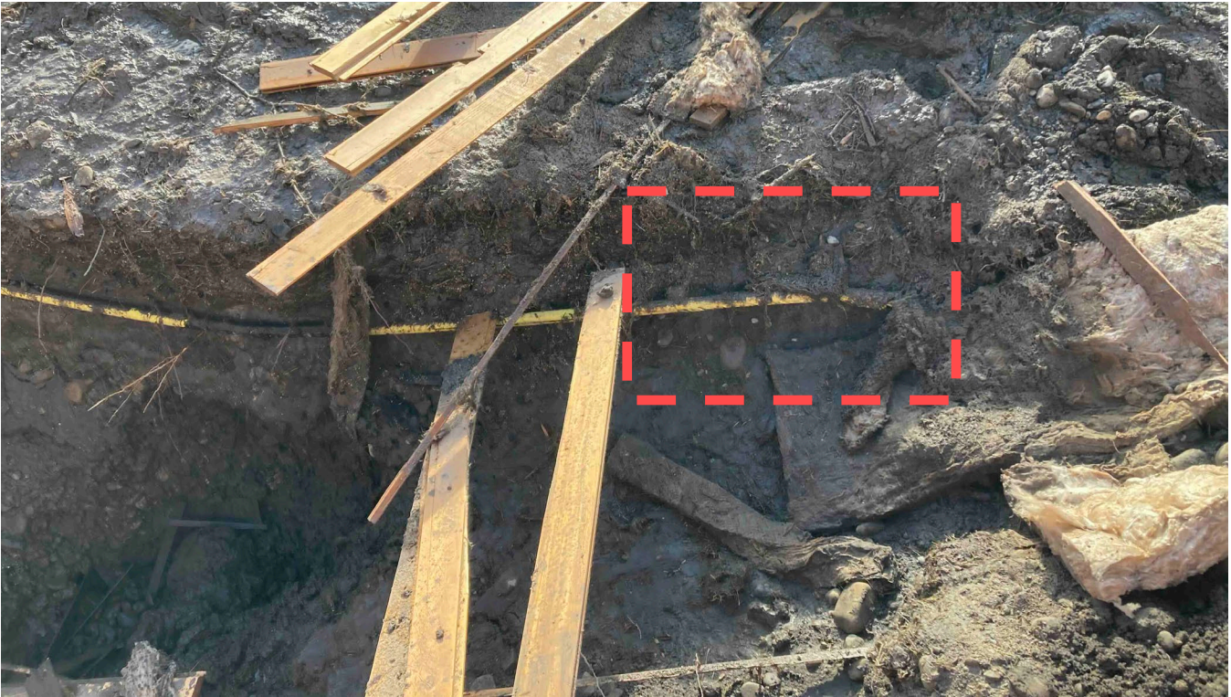
Image 5 – Excavation showing exposed yellow 3/4" steel gas line. Red box showing area gas line was struck and pulled upward by excavating machine.
