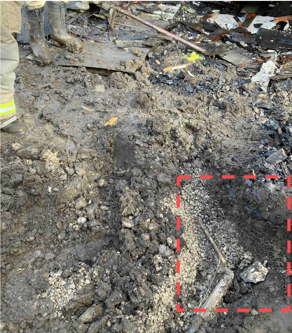
Image 6 – Red box showing area exposed by hand after the incident detecting the separated gas line. 3/4" clear crush backfill was observed surrounding 1/2" plastic gas line.
