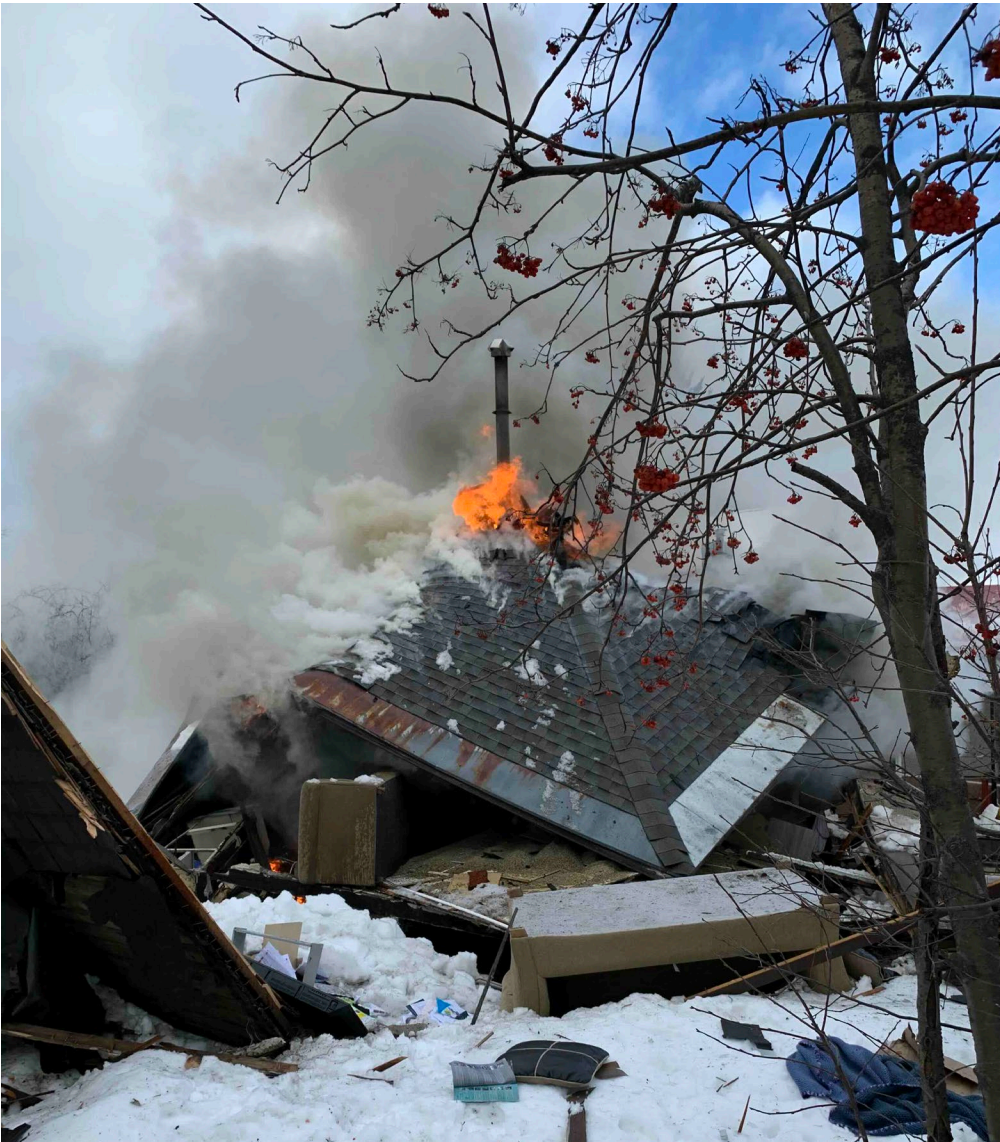
Image 8 – Home collapsed from explosion with fire fueled by leaking gas.
