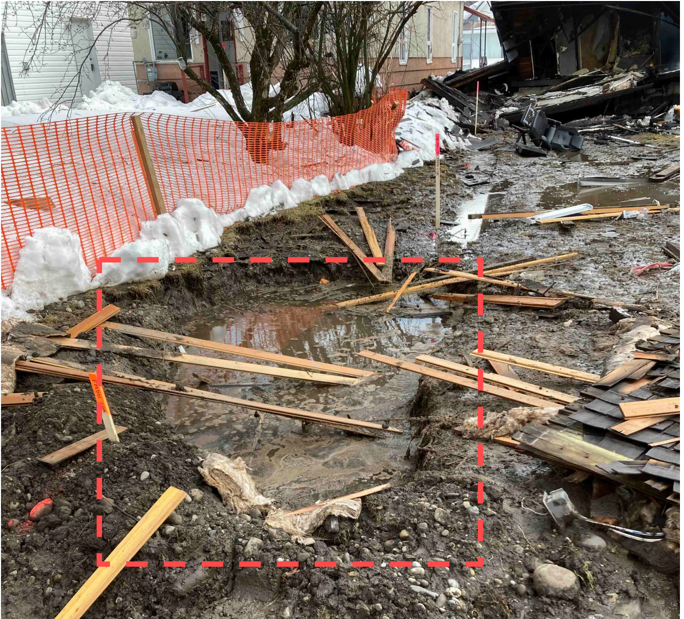
Image 4 – Red box showing area of excavation work and exposed gas line on day of incident. Excavation filled with water after the incident.
