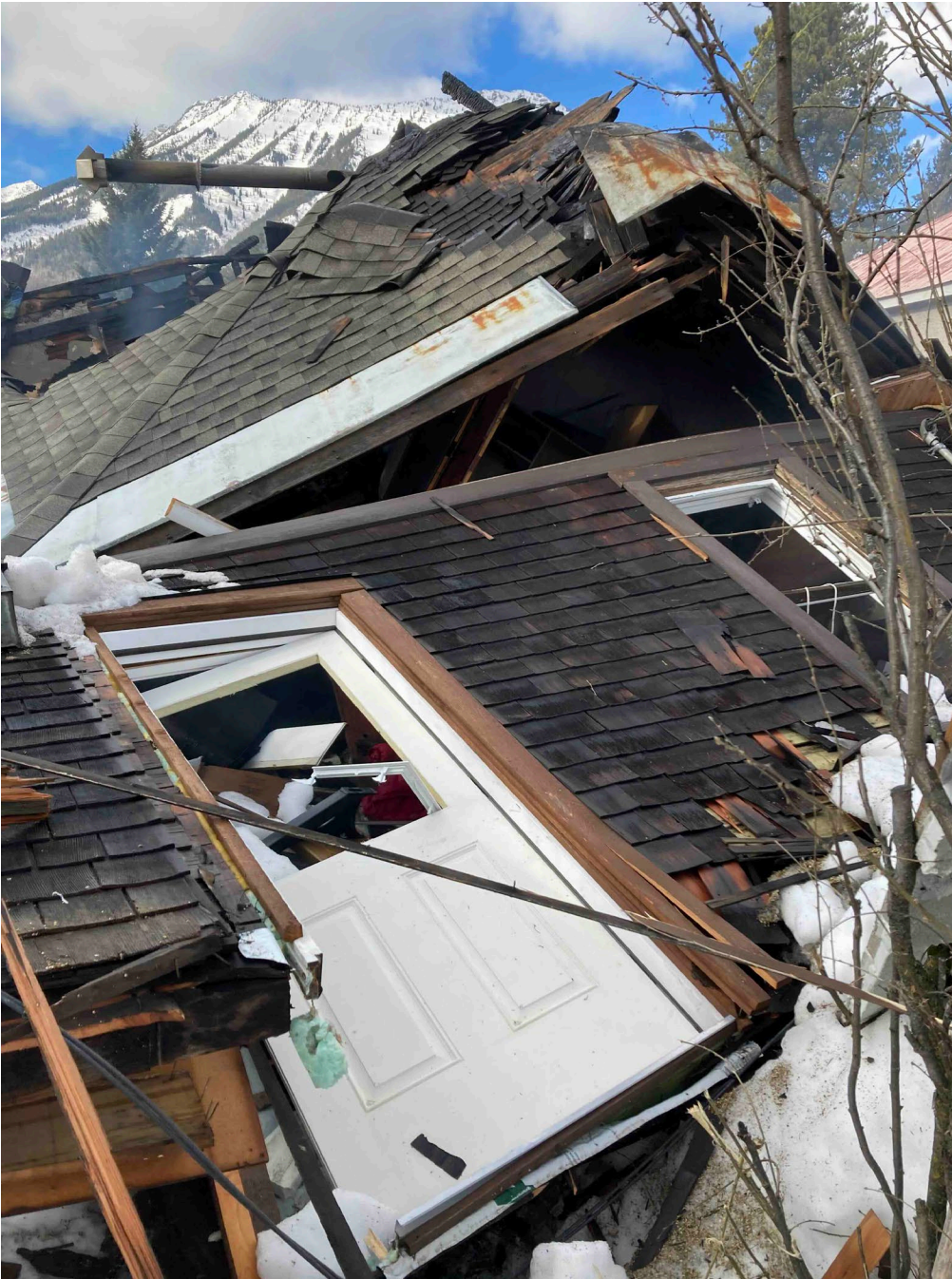
Image 9 - Front of home collapsed from explosion.
