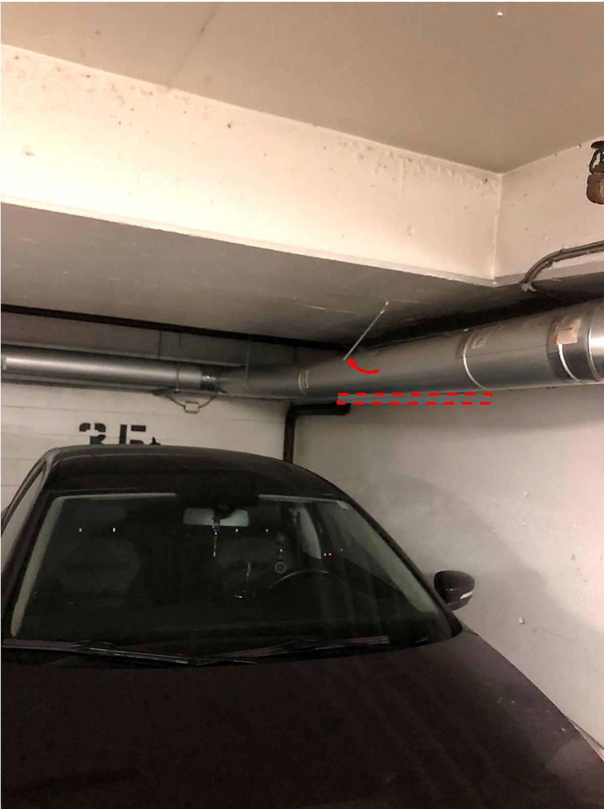
Image 3 - Hanger missing (red rectangle) and rod bent up (red arrow) near missing vent piece.
