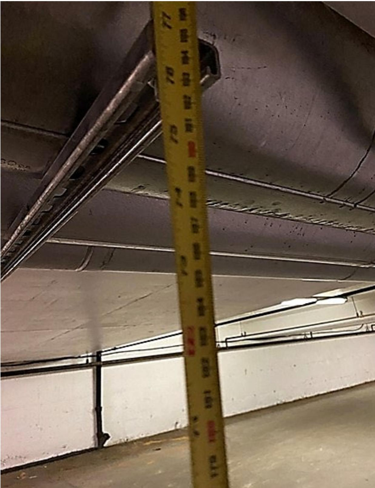
Image 5 - A measurement of 76 inch (6 foot 4 inch) taken by safety officer to the bottom of the vent hanger near to where vent was knocked down.
