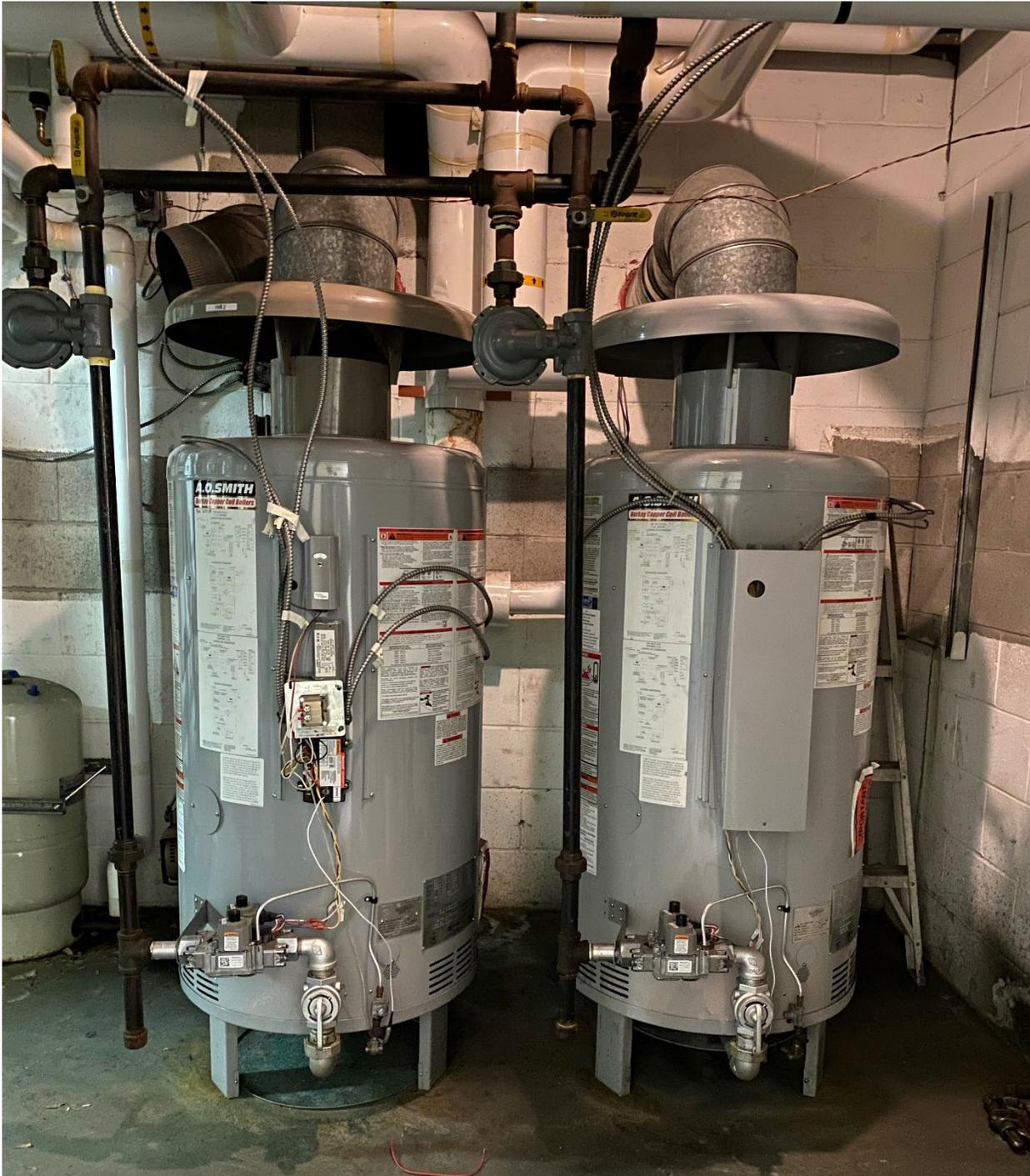
Image 1 - Gas fired water boilers
