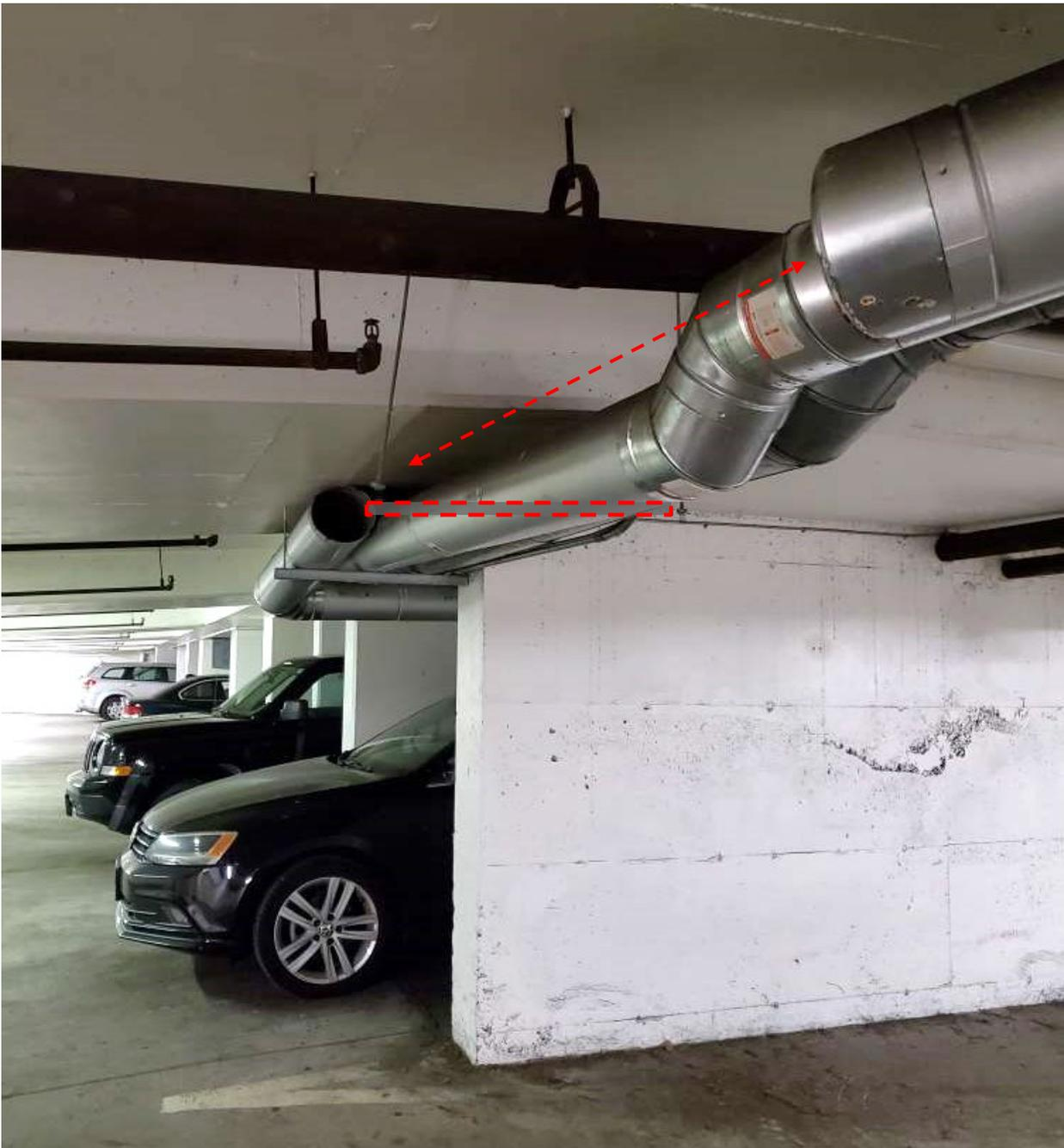
Image 2 - Vent piece down (red arrow) and hangers for vent gone (red rectangle).
