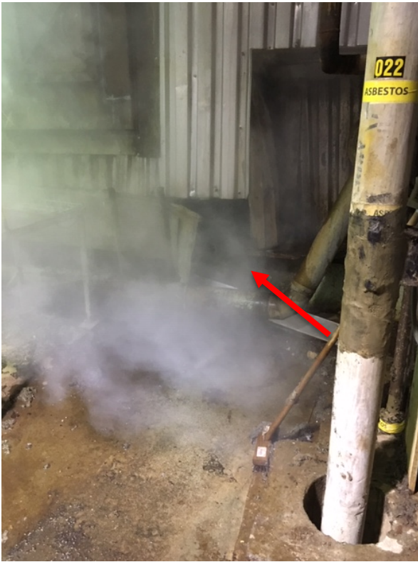
Figure 4: Damaged insulation and cladding following the failure.
