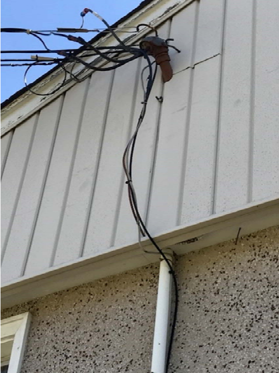
Close up of power conductors, cablevision and Telus communication cable intertwined around service head
