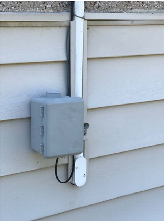
New (black) fibre optic cable connection into existing CATV connection box
