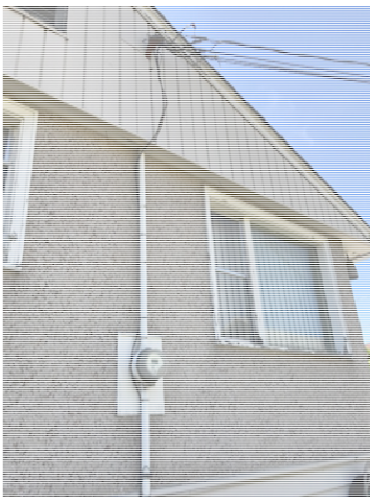
Photo of aerial conductors gathered at same connection point on home. The communication cables are intertwined with the power conductors
