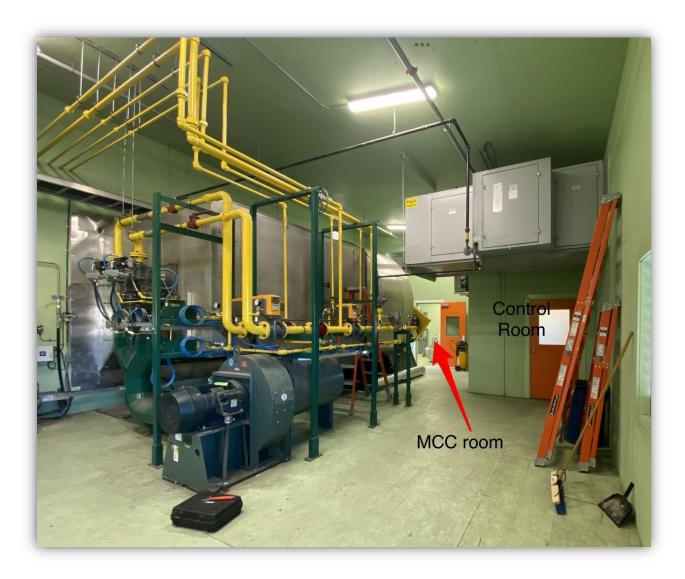
Image 3 – Kiln burner, control room and motor control room adjacent to lumber kiln.
