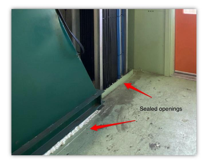
Image 5 – Openings in occupied space CO may have entered through that were sealed after the incident.
