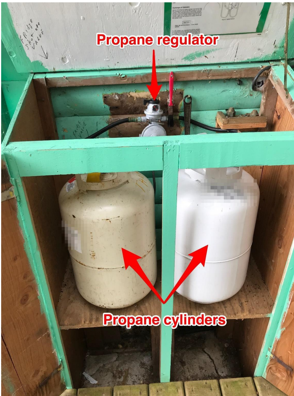
Image 5 – Propane cylinders and regulator installation on side of cabin
