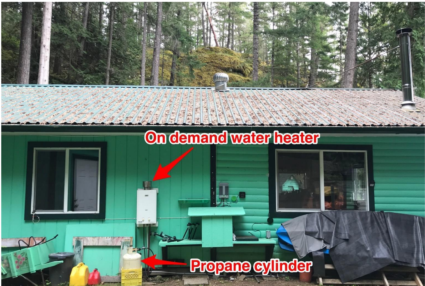
Image 3 – Water heater location on exterior of cabin away from opening windows
