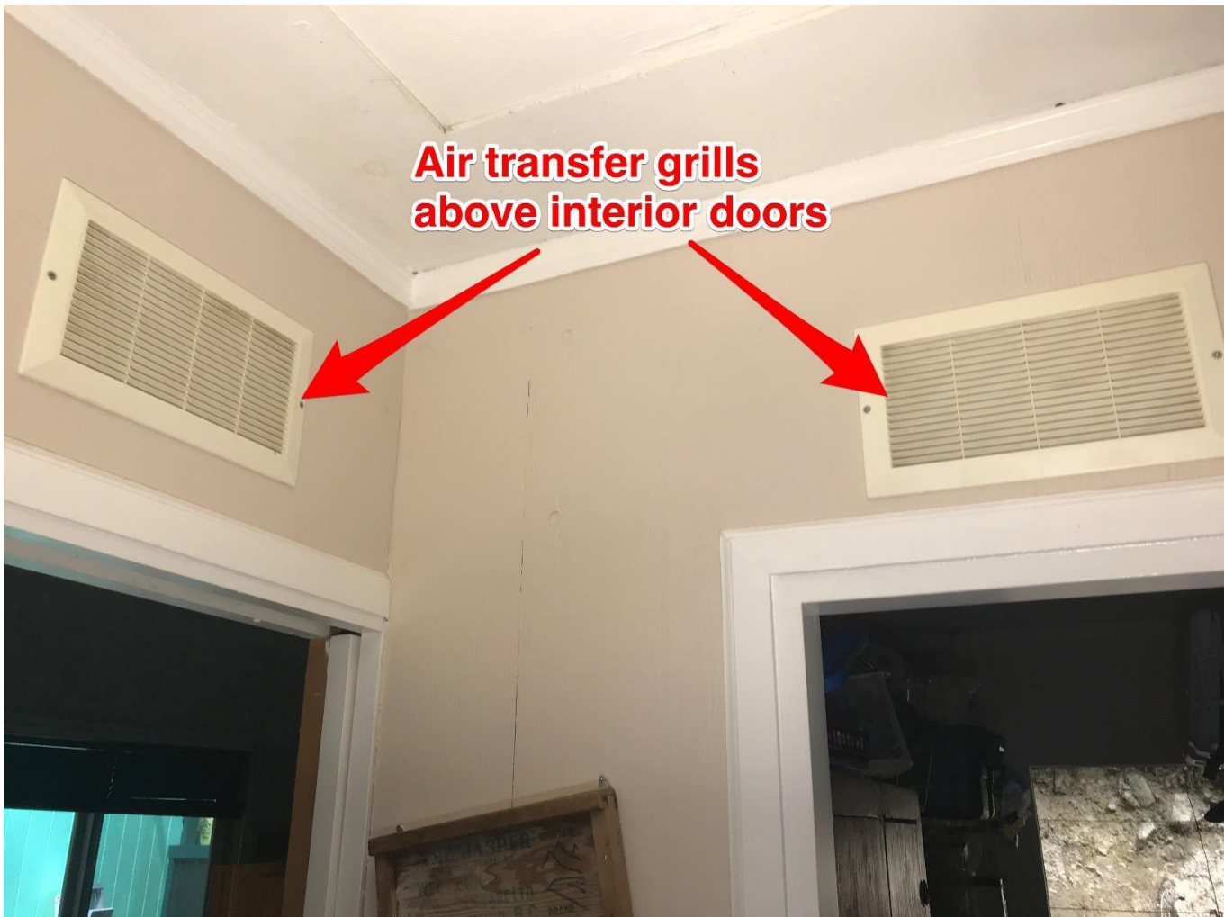
Image 9 – Air transfer grills that are installed above all the interior doors allowing for air to circulate through the cabin
