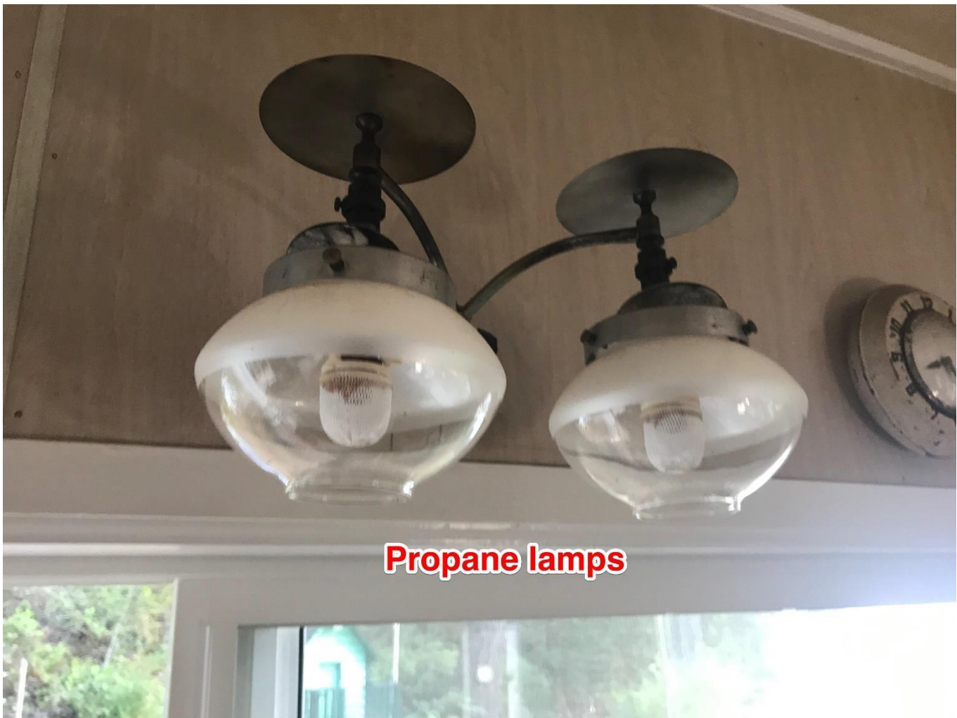
Image 7 – Propane lamps installed in kitchen above sink
