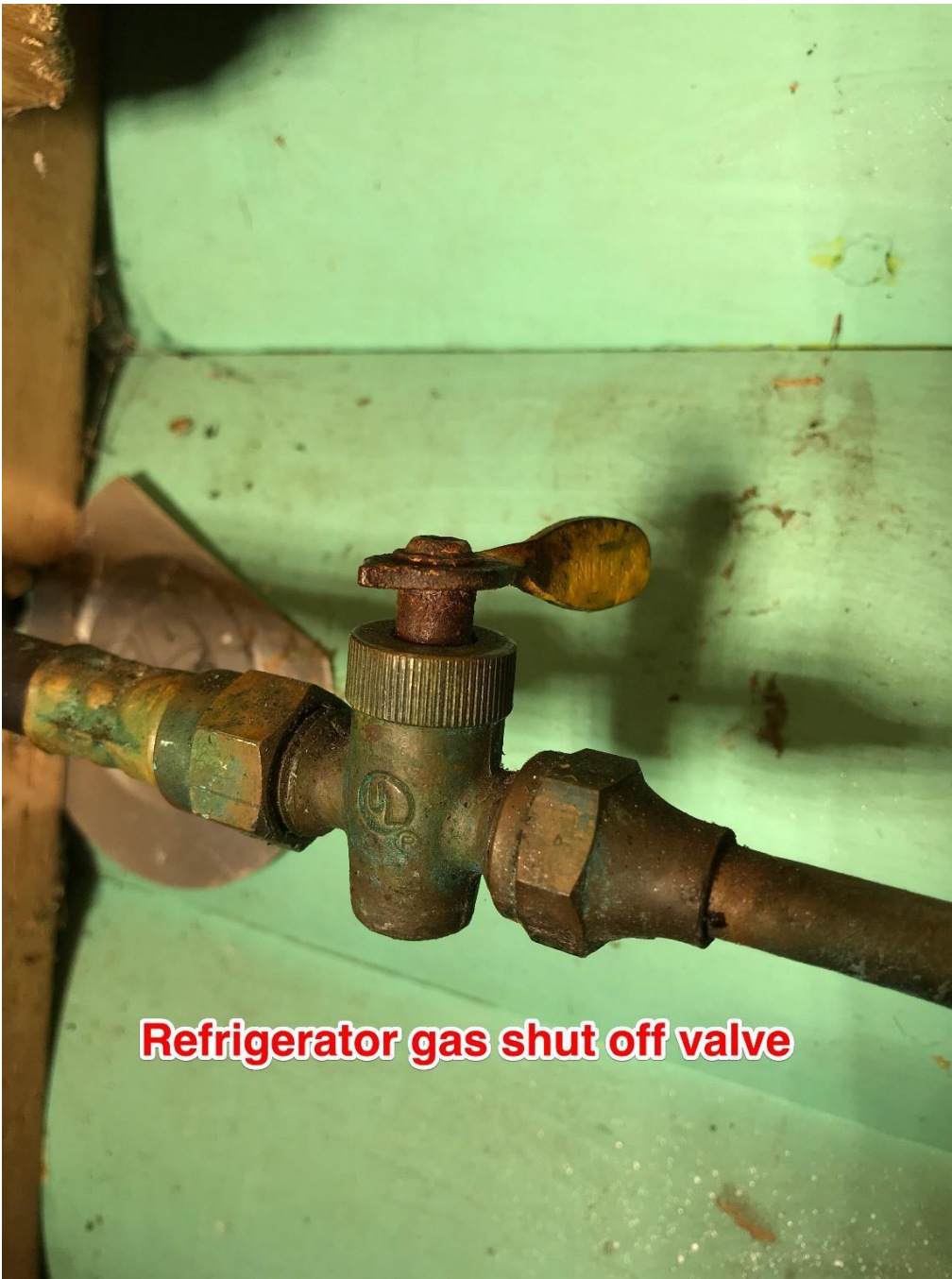
Image 6 – Gas shut off valve for refrigerator installed under propane cylinders
