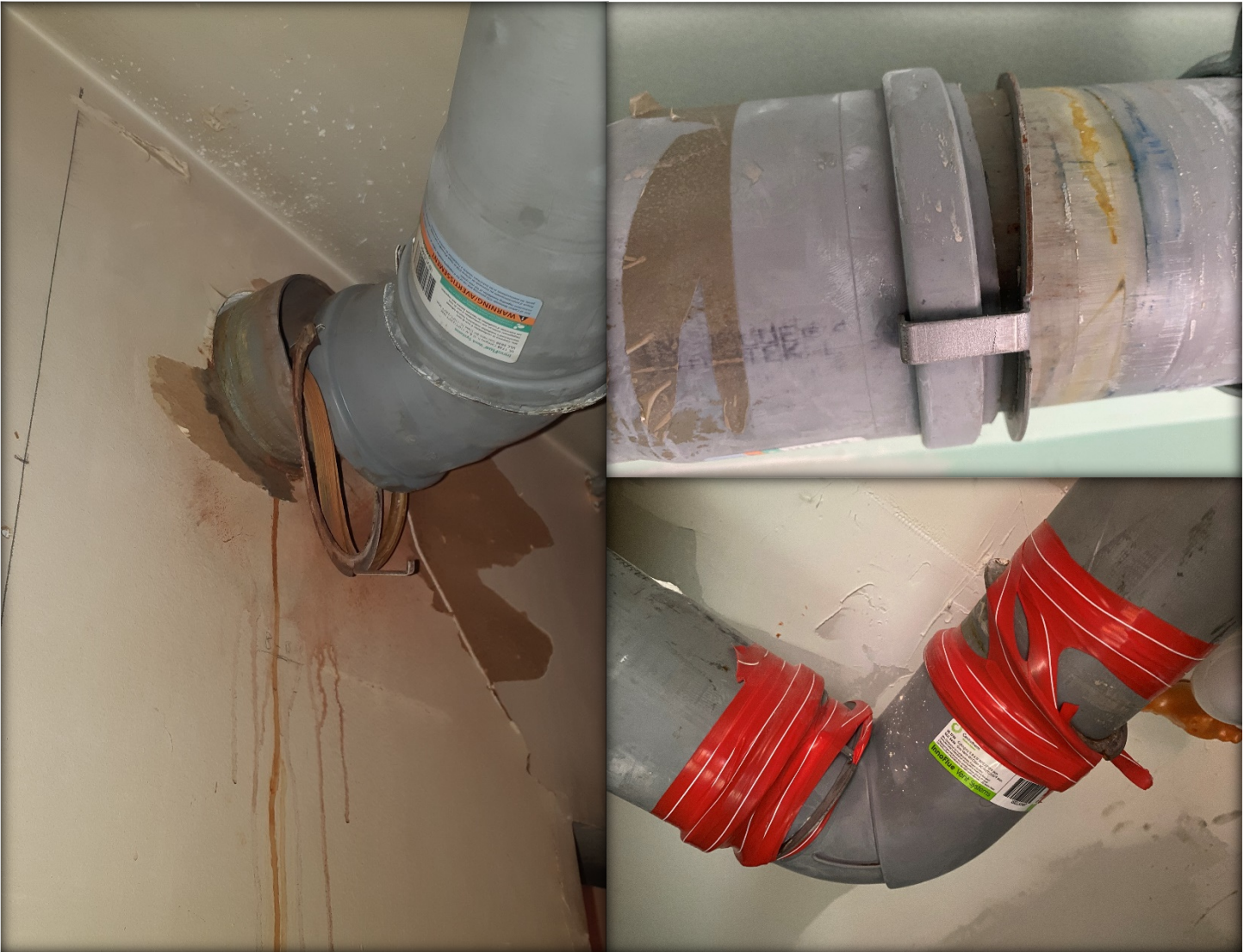
Image 4a, b, c – Boiler venting disengaged from delayed ignition detonations and with improper tape repairs.
