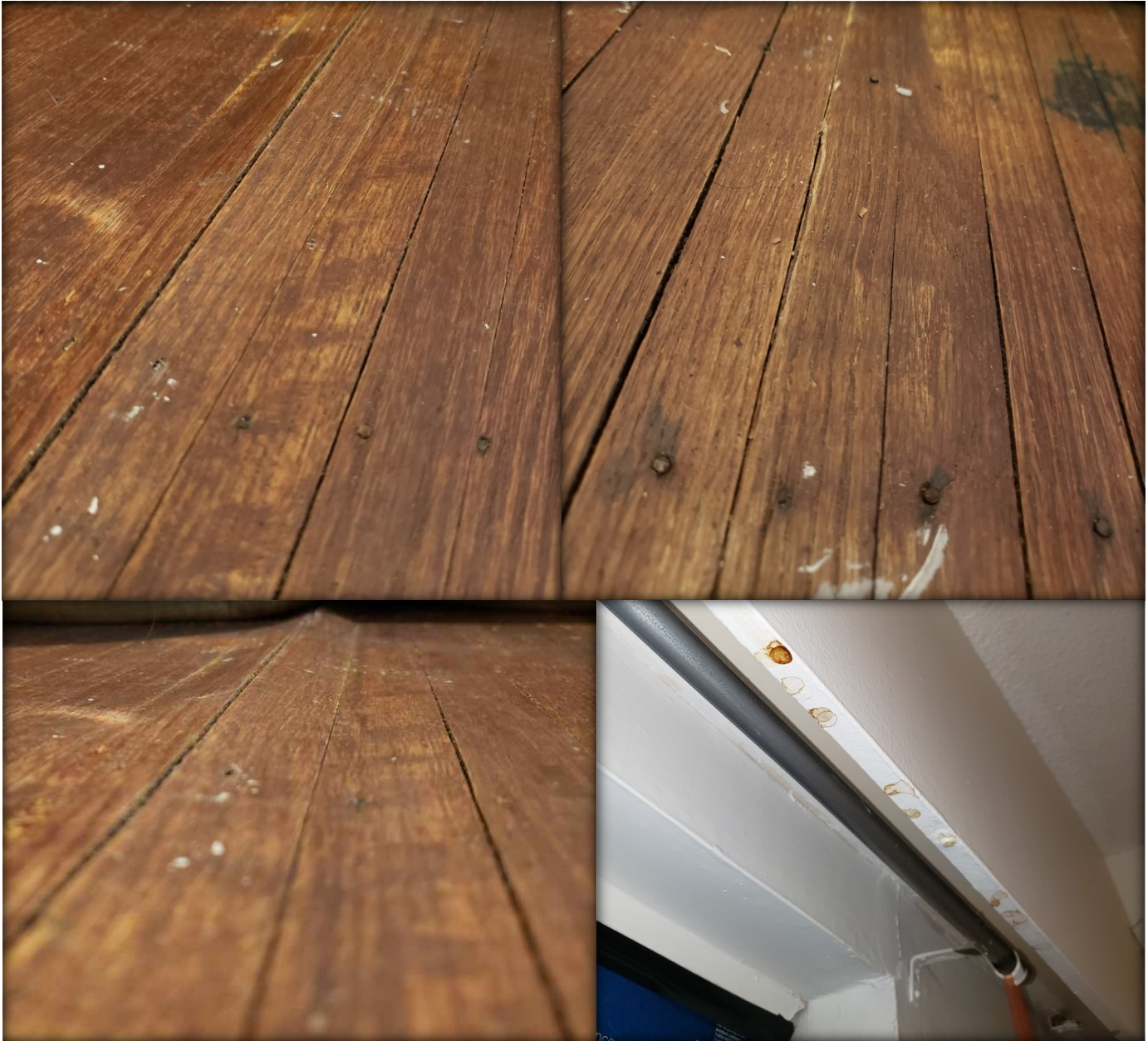
Image 7a, b, c, d – Residence flooring bowed from rising products of combustion and condensate moisture; condensation drops on the ceiling of the residence above the electrical room.
