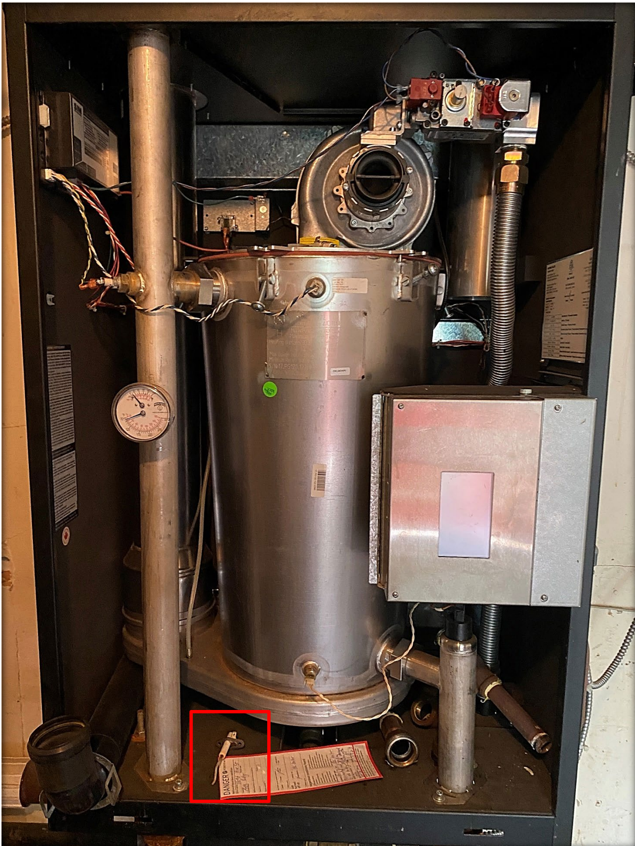
Image 3 - Hydronic boiler. Note the extra used single prong ignitor in the red rectangle.
