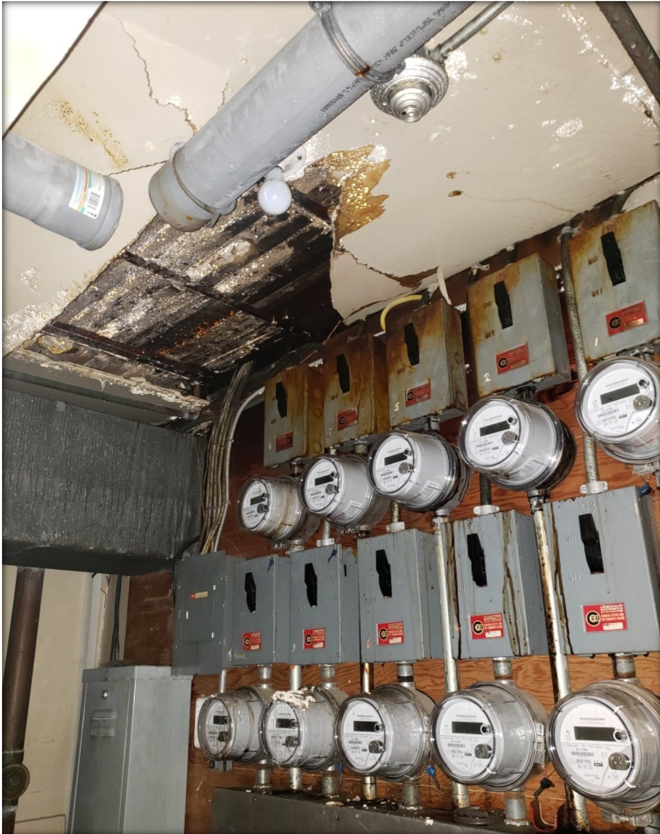
Image 6 - Photo from Nov 2020 showing damage from products of combustion and condensate to the electrical room ceiling/electrical equipment and the corner vent piece fallen from explosive detonations.
