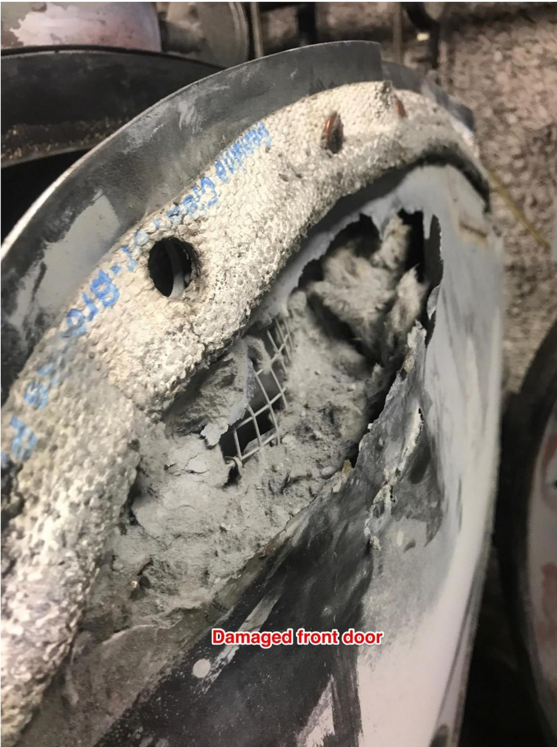
**Image 7 -** Damage to boiler front door
