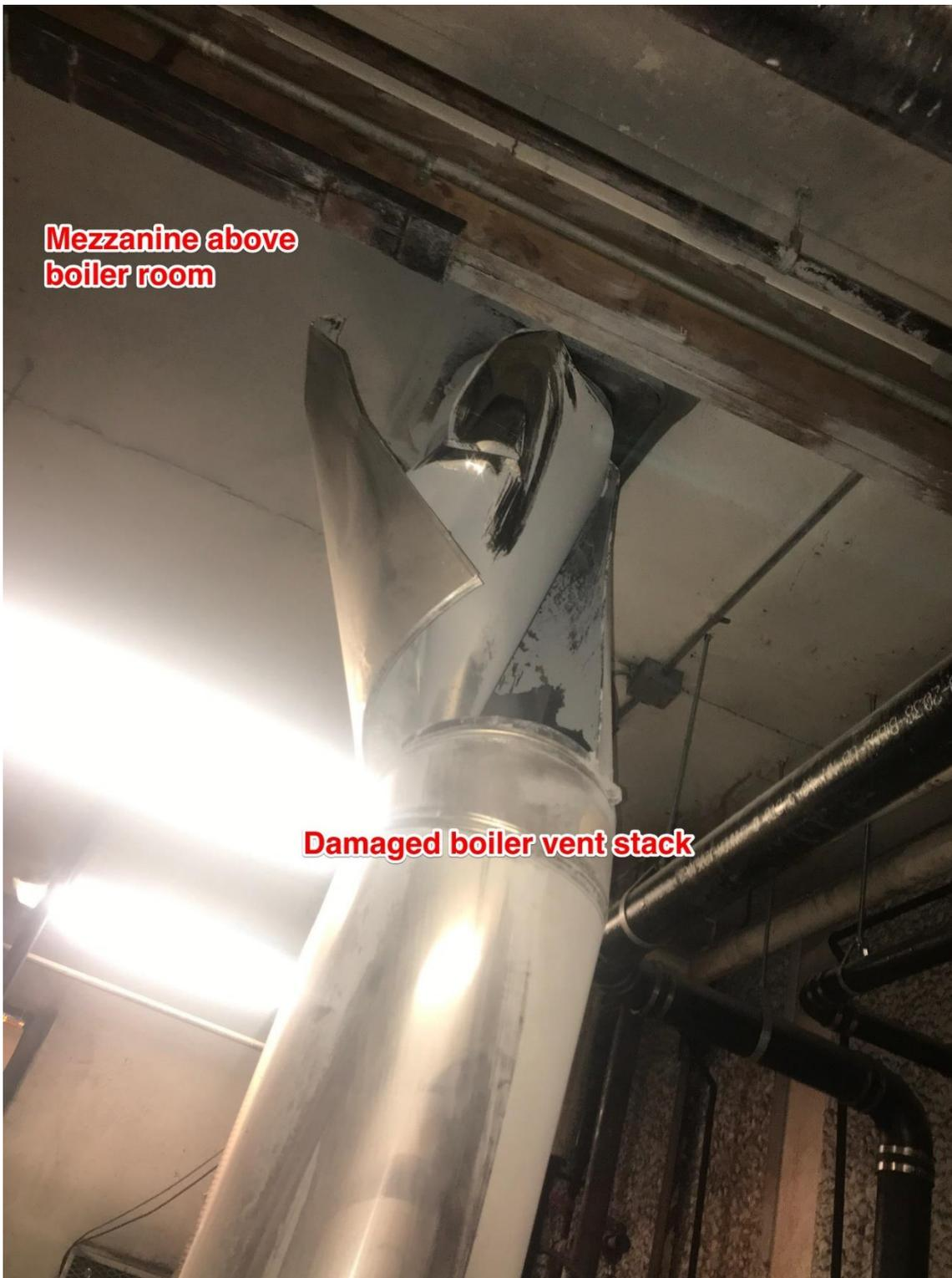
**Image 4 - Boiler vent stack above boiler**
