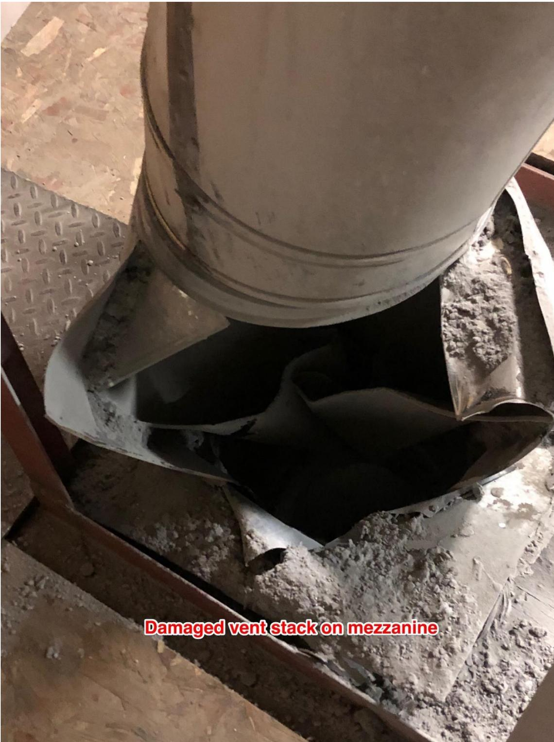
**Image 5 - Boiler vent stack at mezzanine above boiler room**
