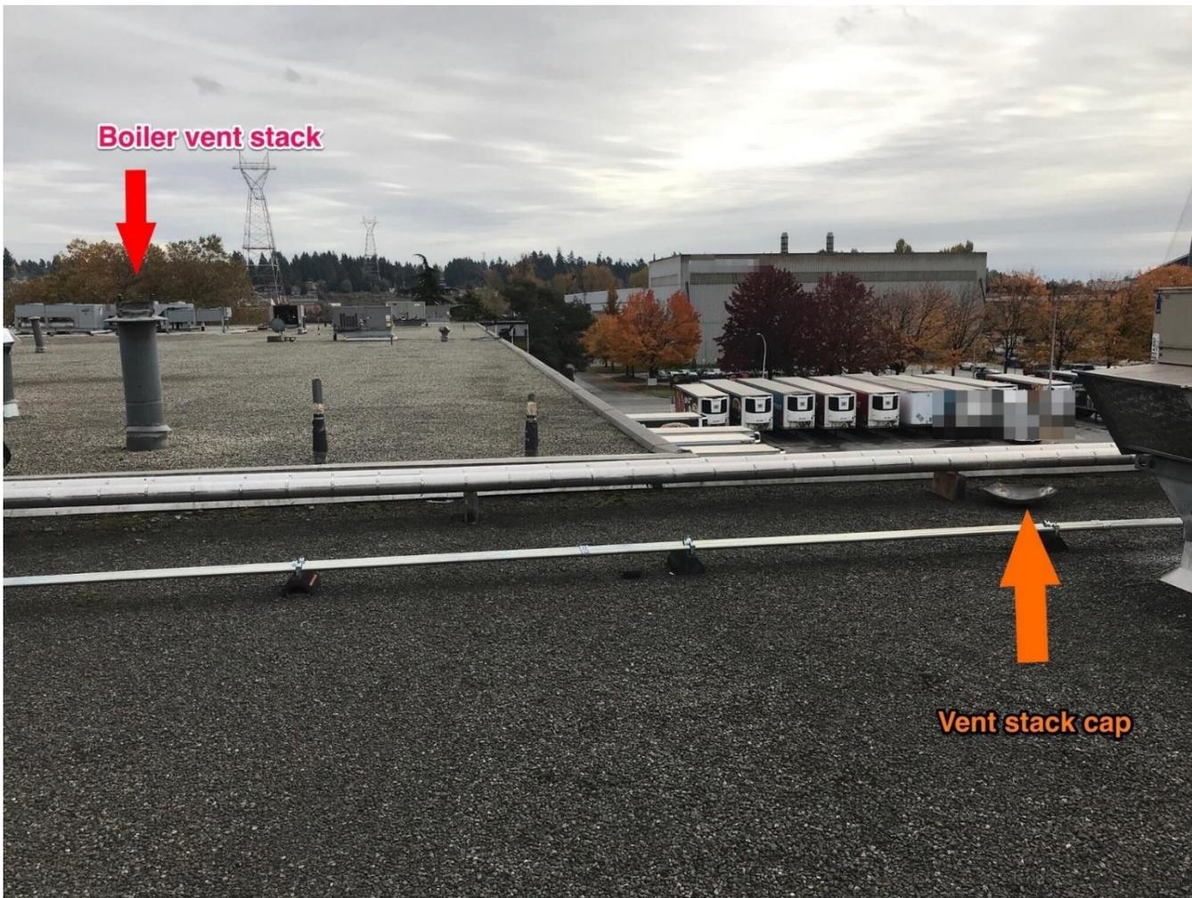
**Image 6** - Location of vent cap after it was blown off the boiler vent stack by the explosion
