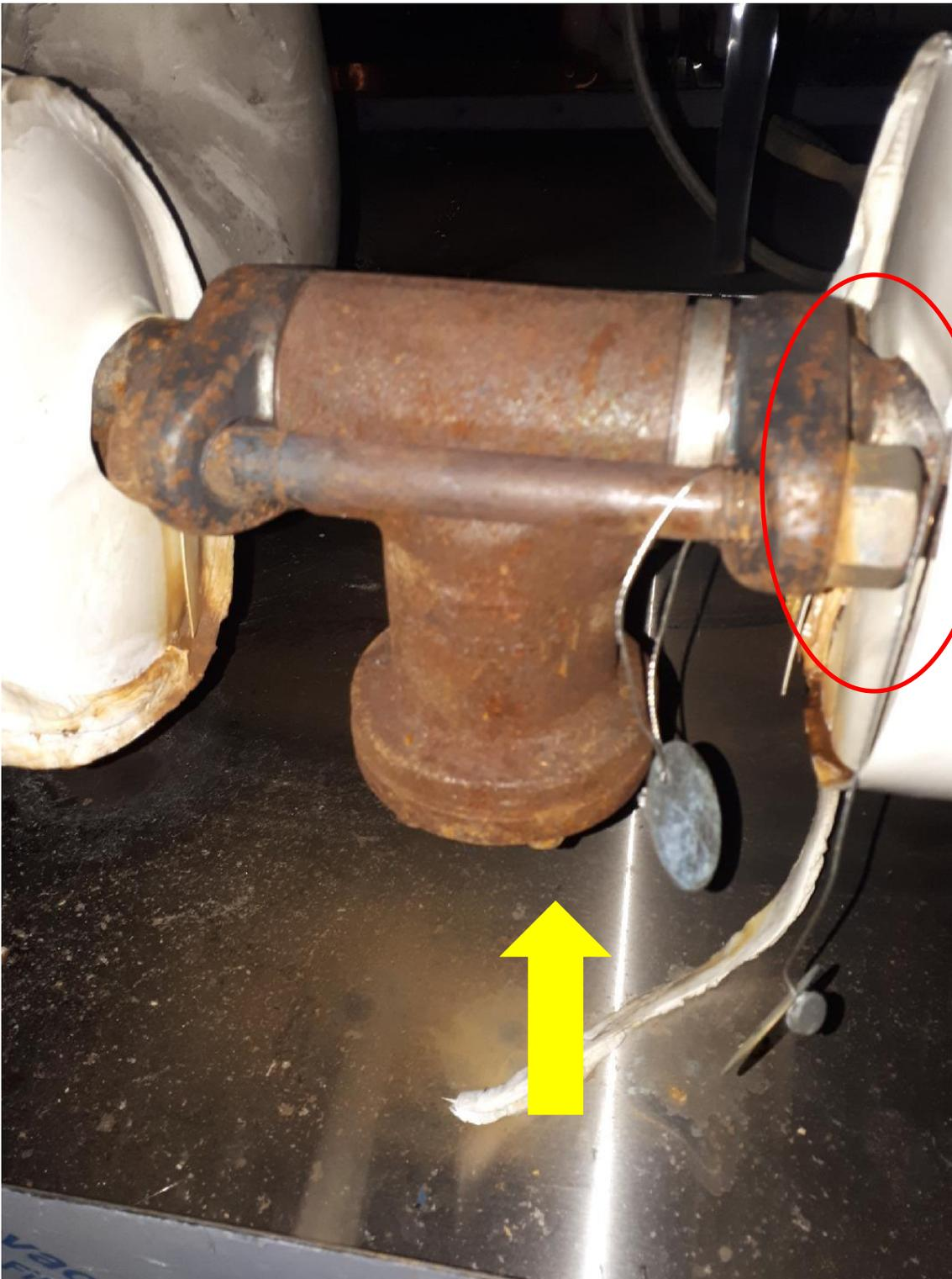
Photo 2 (Submitted by client) Shows the ammonia strainer (yellow arrow) and the flange where the gasket was located (red oval)
