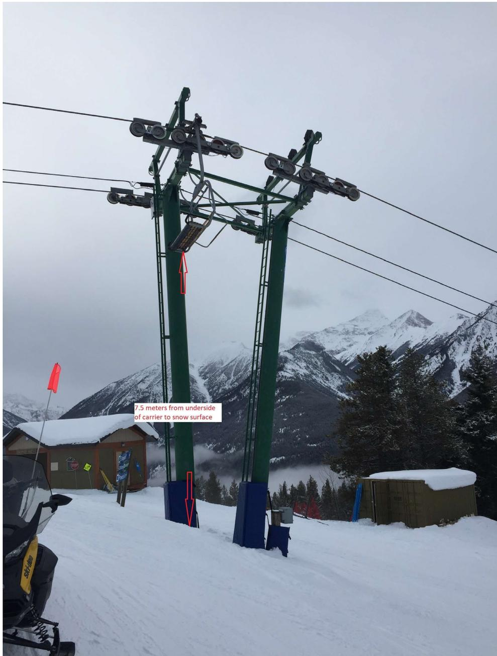
Image - Carrier position at time of fall. 7.5 Meters from underside of carrier to snow surface
