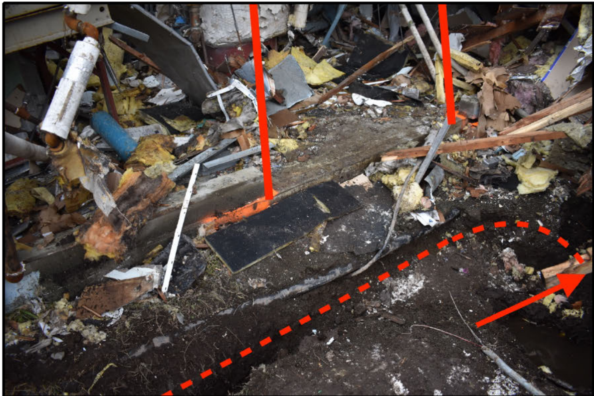
Figure 2: Shows area of exterior to the mechanical room. The vertical lines indicate the open doorway, the dashed line shows the natural line and the arrow indicates the approximate location of the break in the natural gas line.
