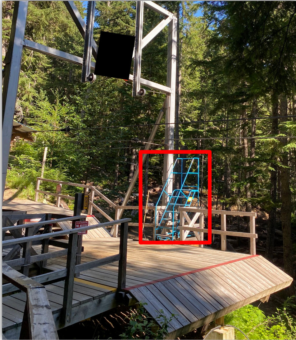
Image 4 – The third zipline’s landing platform. [RED] Blue rolling staircase in the safe stored location on the rider’s right side.
