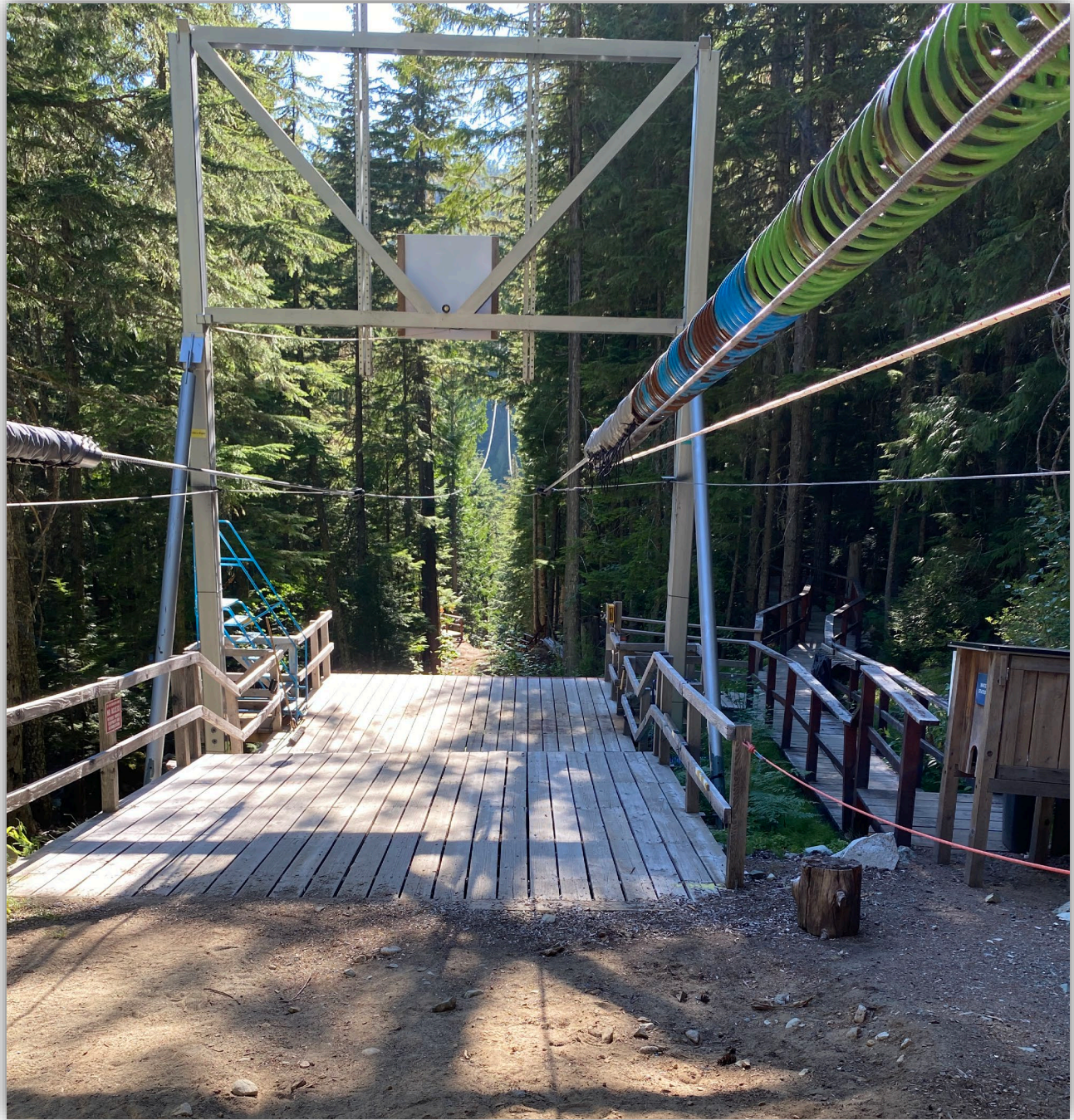
Image 5 – Third zipline landing platform showing braking mechanism.
