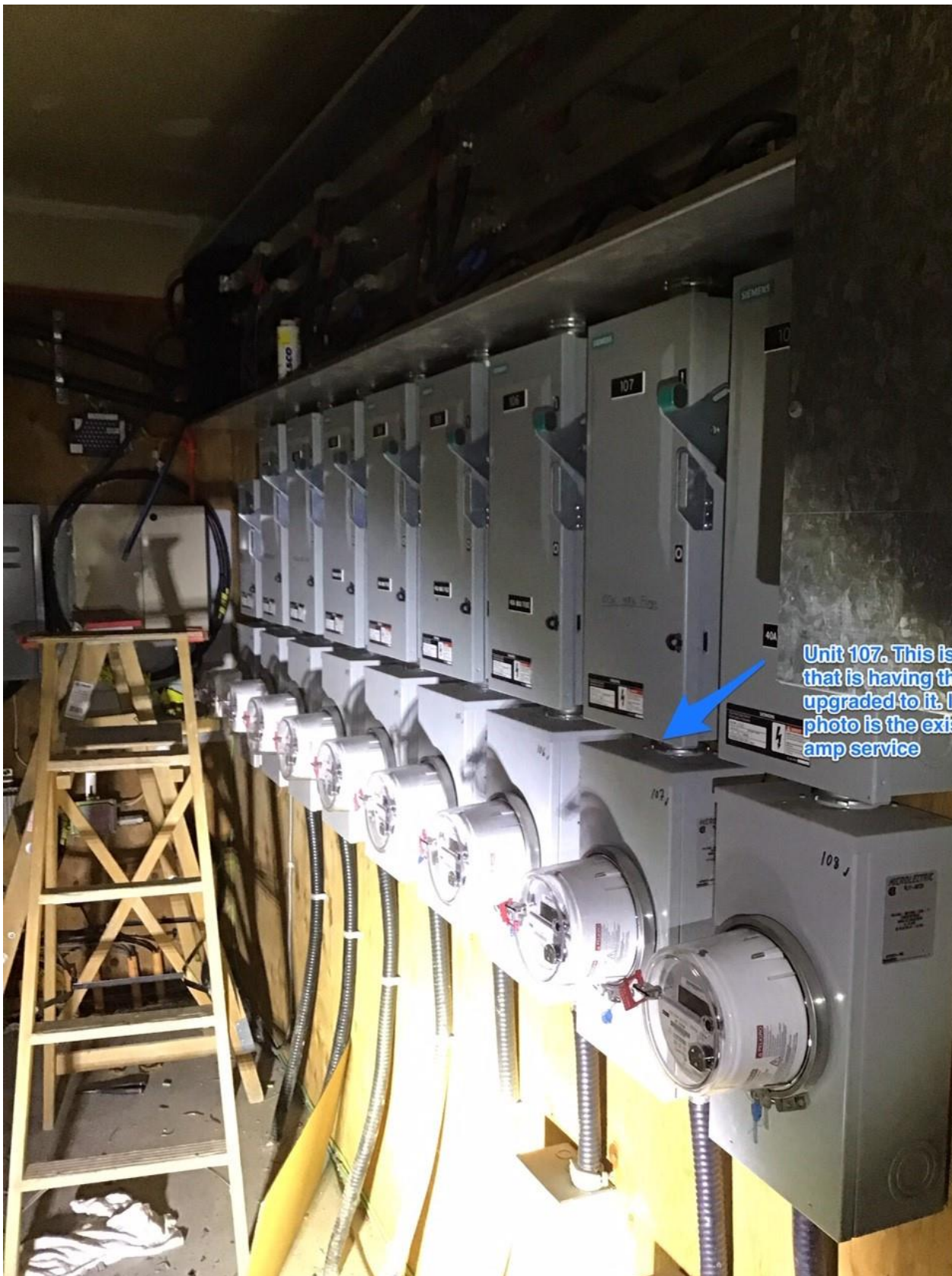
PHOTO 1: All of the fused disconnect switches above the meters were found in the on position.
