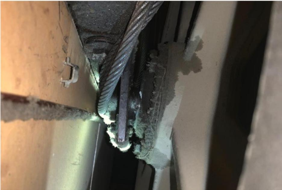
**Photo 3** – 3 loose ropes on the side of the Deflector Sheave
