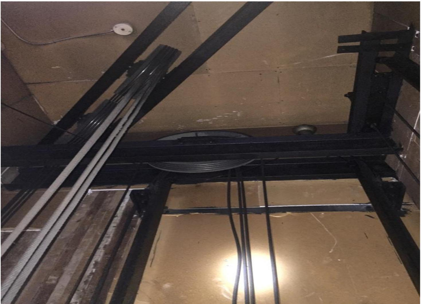
**Photo 9-** The three deflector sheaves mounted at the top of the hoistway. The sheave mounted furthest to the back wall is the sheave with the damaged bearings. Three ropes hang loosely to the side of the sheave while one remains in the groove.
