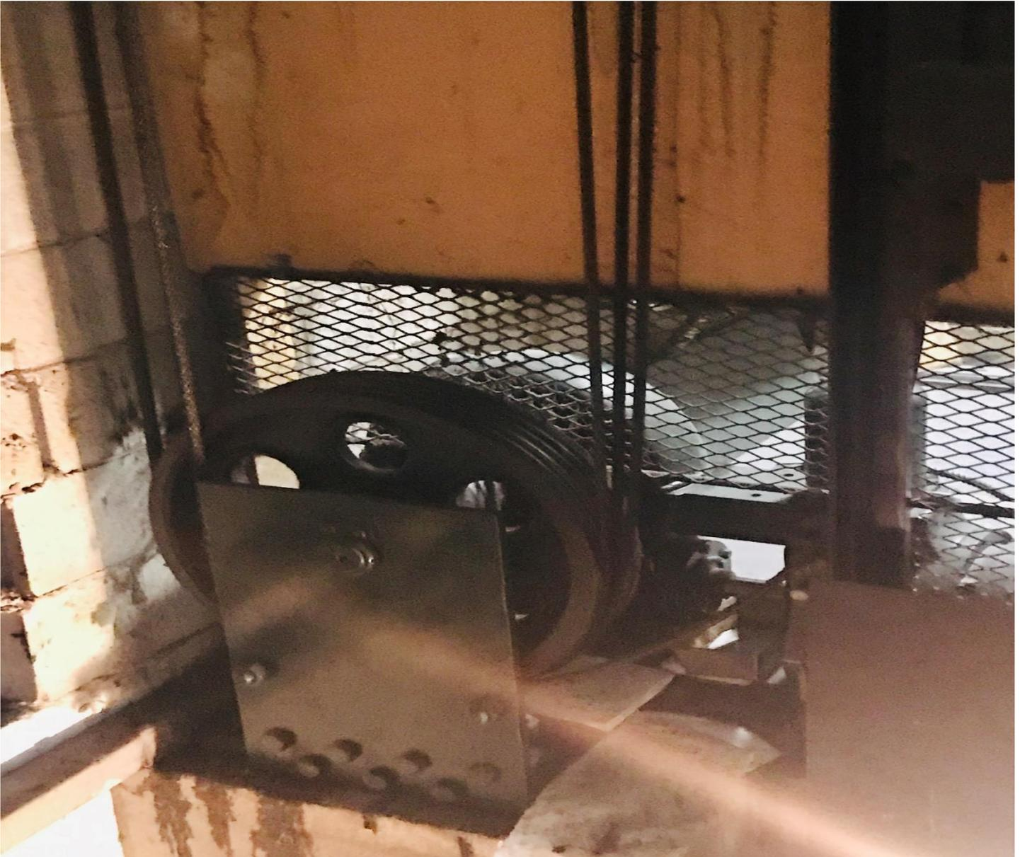
**Photo 10-** The traction elevator machine located in the basement. The drive sheave is positioned inside the hoistway while the motor end sits in the machine room. The ropes can be seen hanging loosely.
