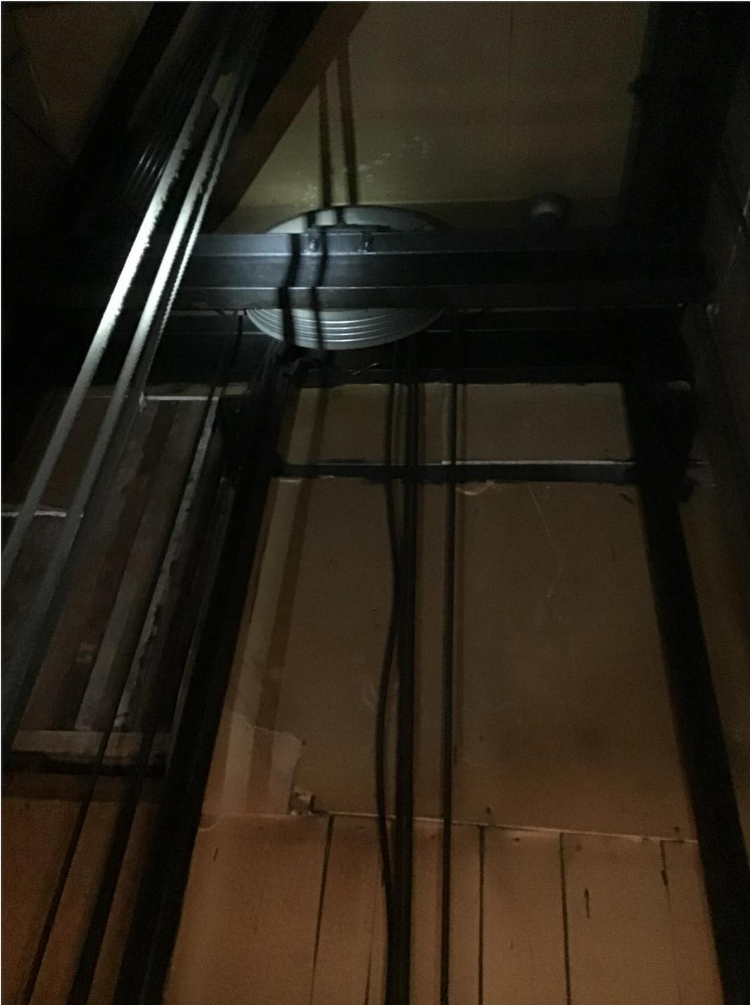
**Photo 5** – showing the Overhead Deflector Sheave with only 1 rope in place, others hanging loosely.
