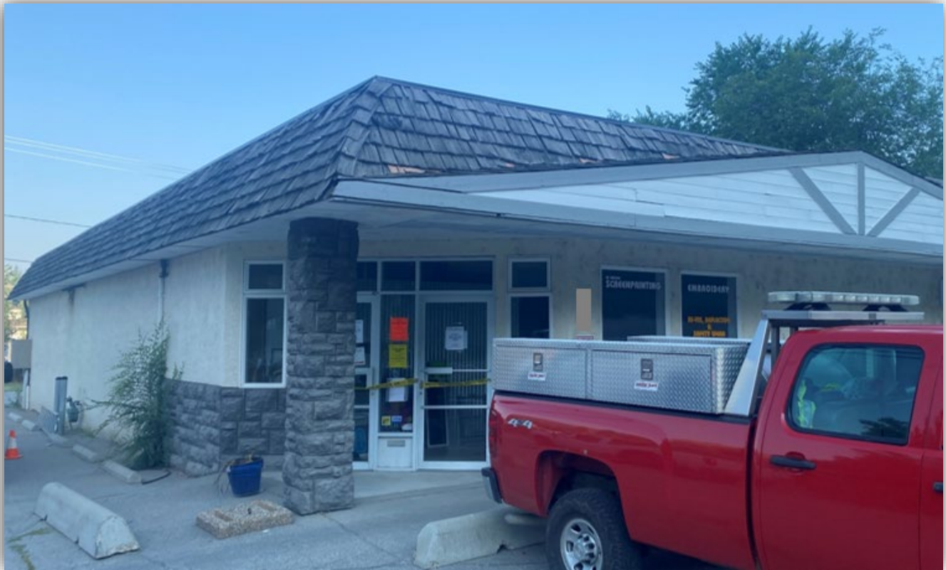
Image 1 – Front of the building housing the textile dryer that exploded.
