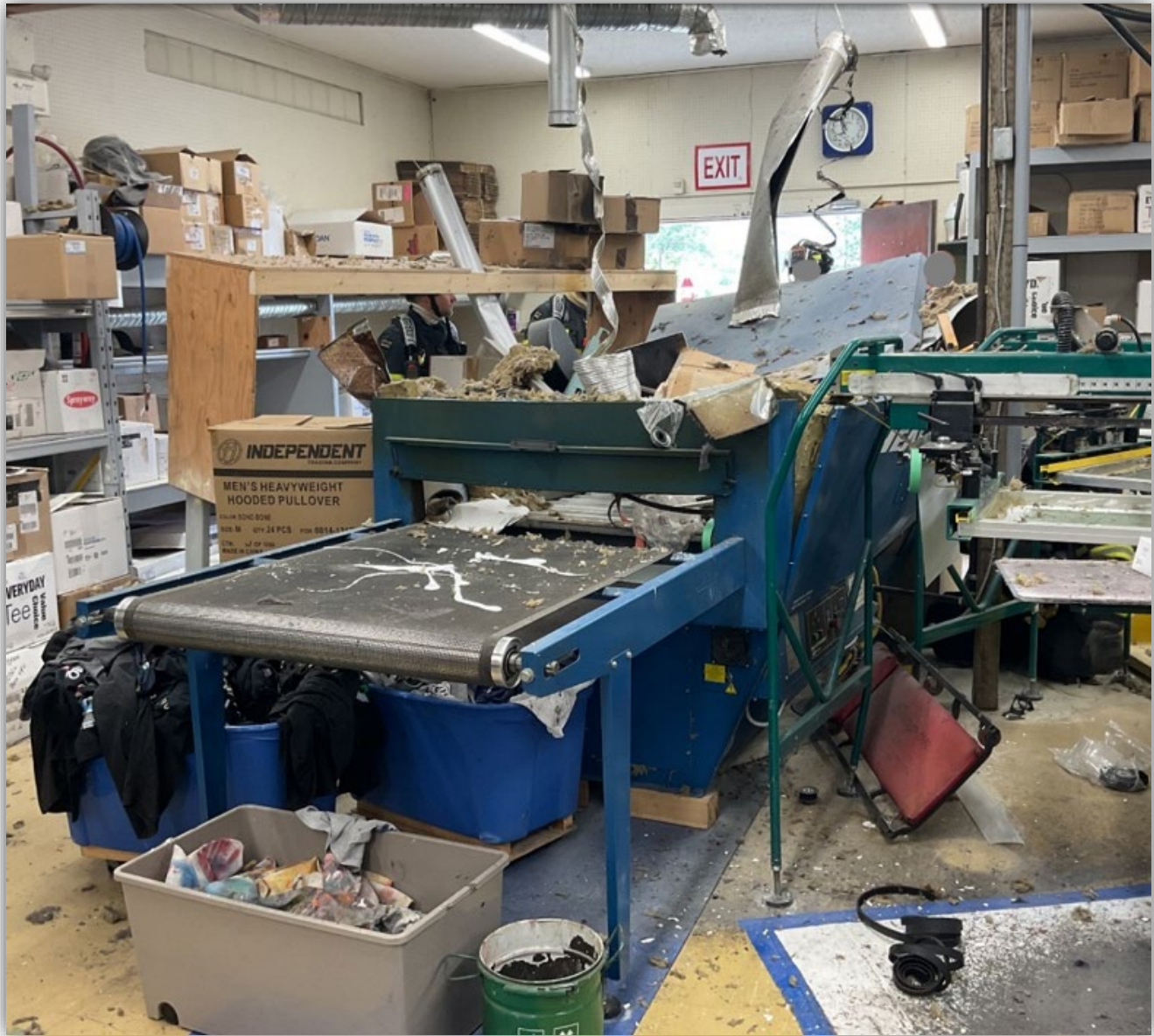
Image 2 – The textile dryer after the explosion showing the pushed-out dryer panels and explosion debris.
