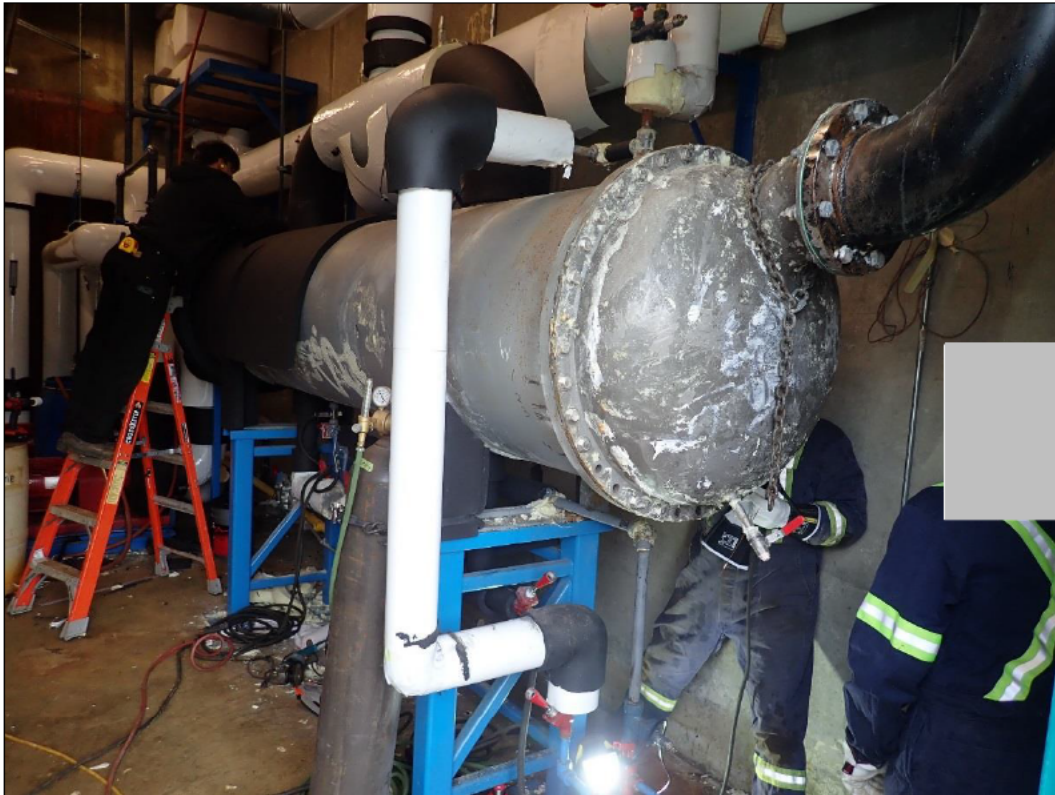
Figure A-1 Overall view of stripped chiller. Heads are titanium alloy.
