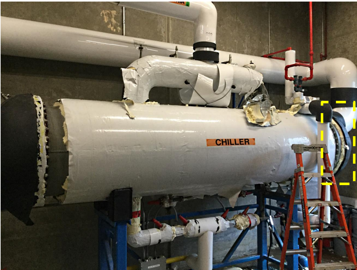
Figure 2: Location of weld failures along 180° of the circumferential shell to head flange weld.
