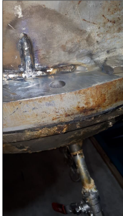
Photo B-6: Location #5 final root pass inspection.
