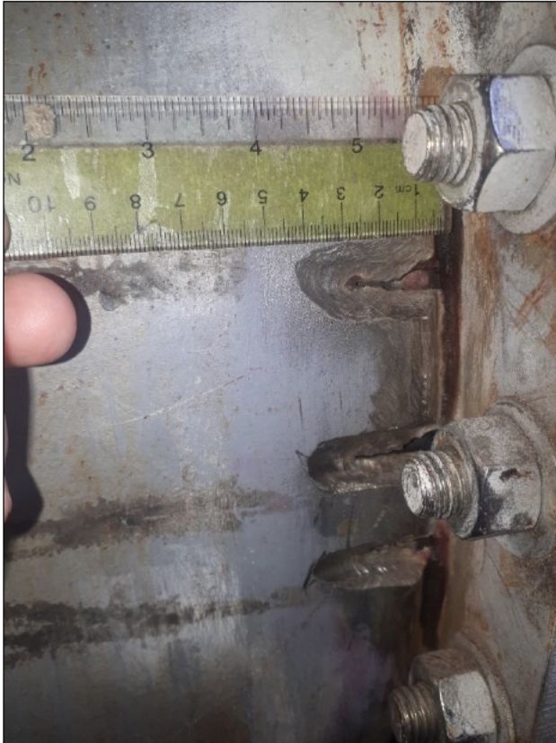
Photo B-5: Close-up of typical excavation site with fillet removed.
