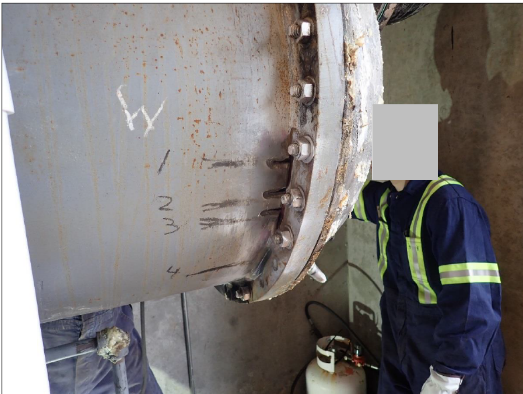
Figure A-2 Opposite side of chiller flange showing location of cracks labelled 1, 2, 3, and 4.
