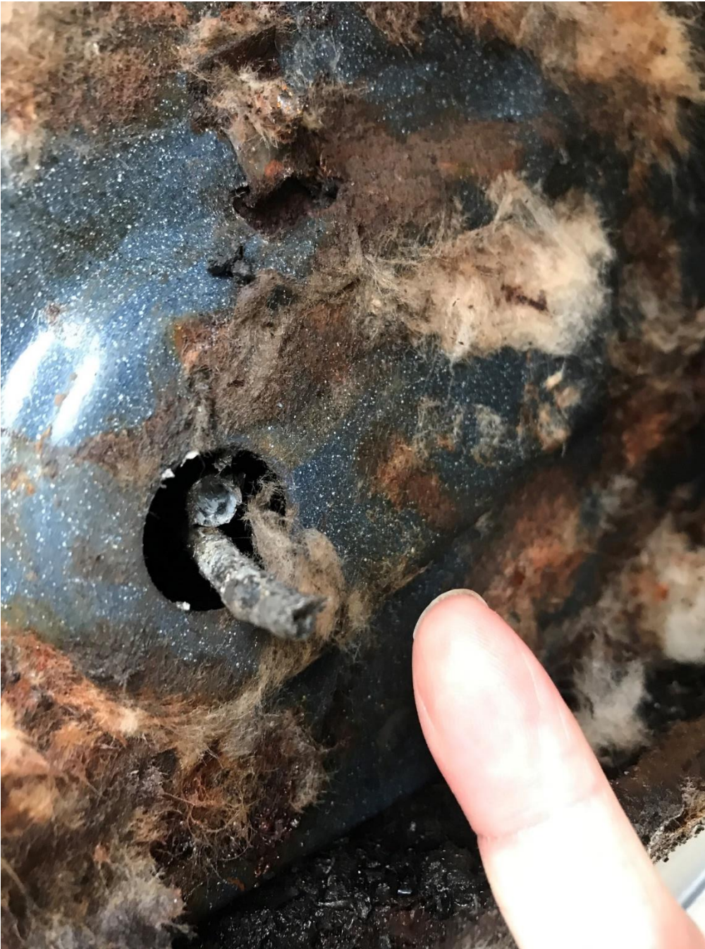
Image 4 - Corroded and plugged lines. Insulation removed for clarity
