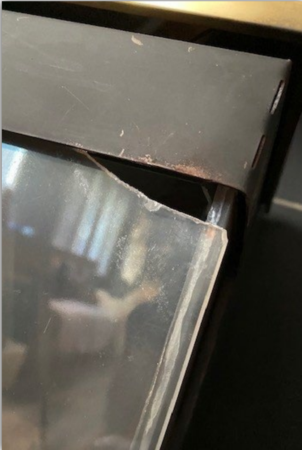
Photo 4 - Front glass panel with damage to glass on top right corner.
