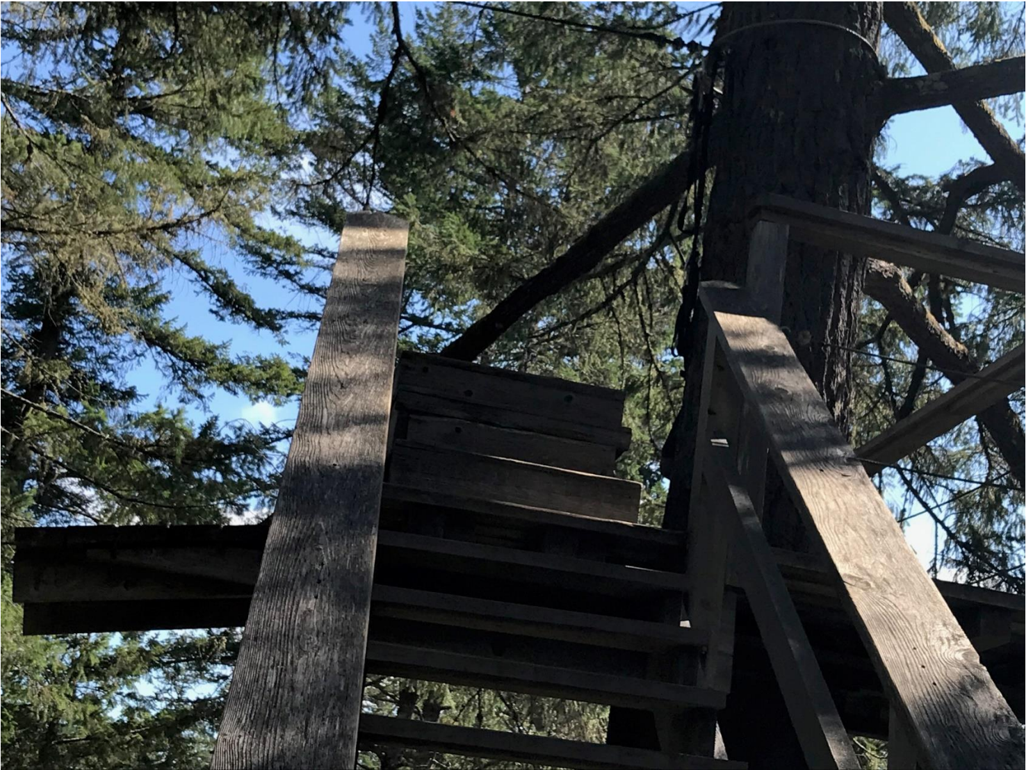
Lower landing platform.
