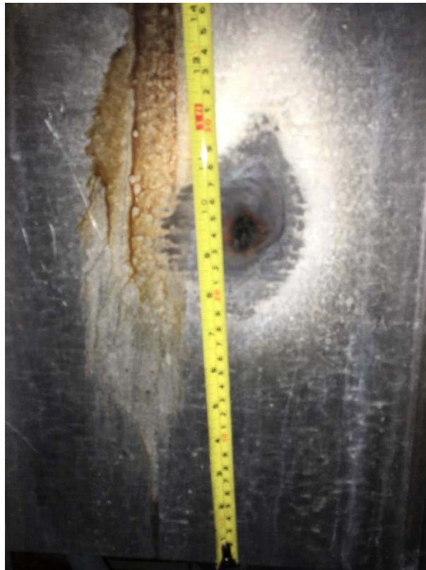
Above & below- hole observed in what appears to be the combustion area in rear side of boiler #1
