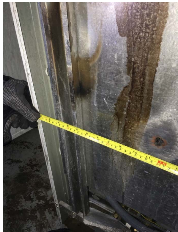
Above & below- hole observed in what appears to be the combustion area in rear side of boiler #1
