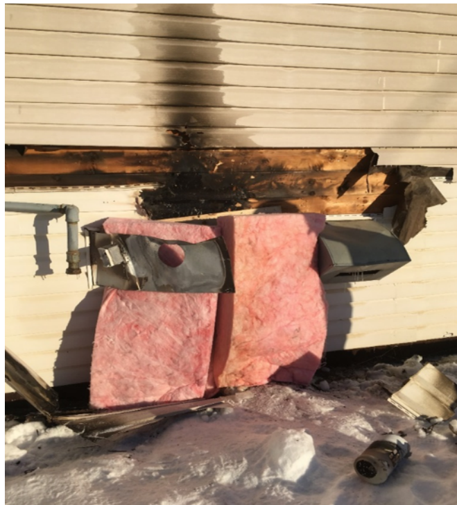
Below-exterior wall damage (insulation placed post fire to keep cold out)
