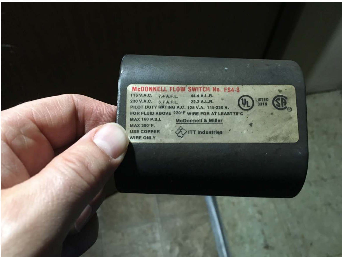
Above -flow switch held by contractor / below - flow switch cover removed by contractor. (wiring in photo above is the low water cut off with cover removed)
