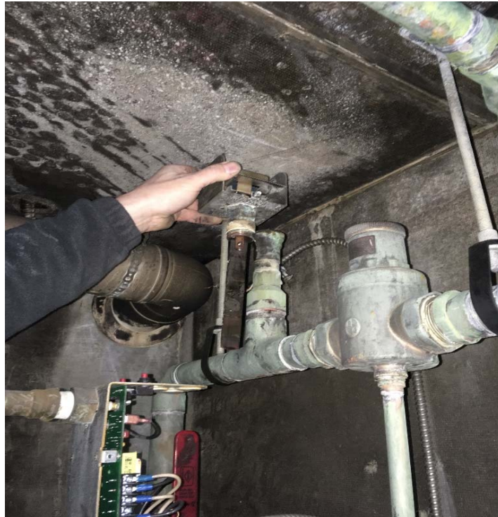
Above -flow switch held by contractor / below - flow switch cover removed by contractor. (wiring in photo above is the low water cut off with cover removed)
