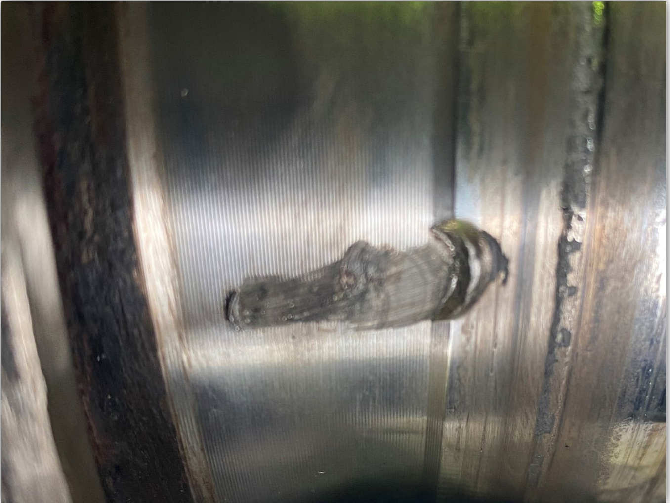
Image 9 - Closeup of alignment flange set screw indentation mark on step-drive main-shaft.
